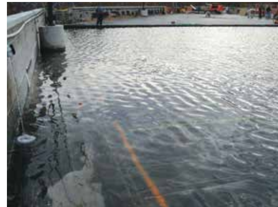
Figure 1. Flood testing a roofing membrane.
