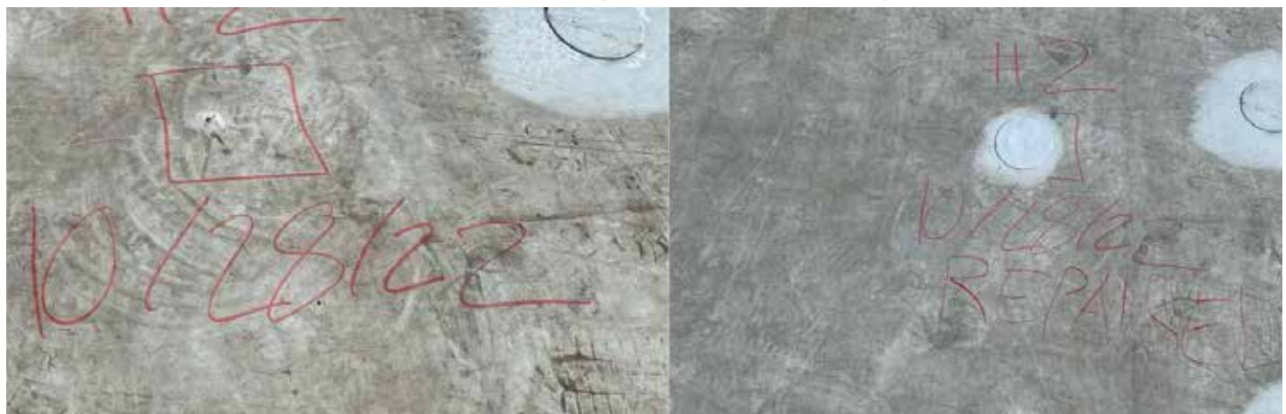
Figure 6. A breach is located and repaired.
