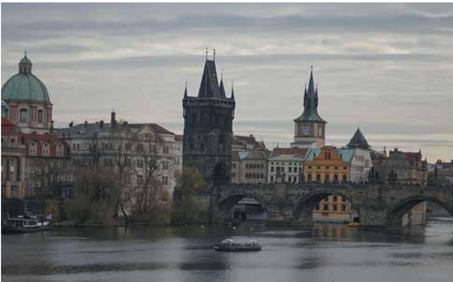
Figure 8. Medieval bridge tower over a river with limited roof access, in Prague, Czech Republic.
