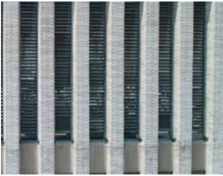
Figure 4. Aerial imagery of the exterior of a masonry-clad parapet.
