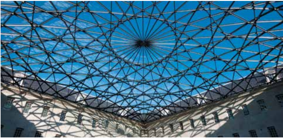
Figure 7. Nonstandard grid shell at Het Scheepvaart Museum in Amsterdam, The Netherlands.
