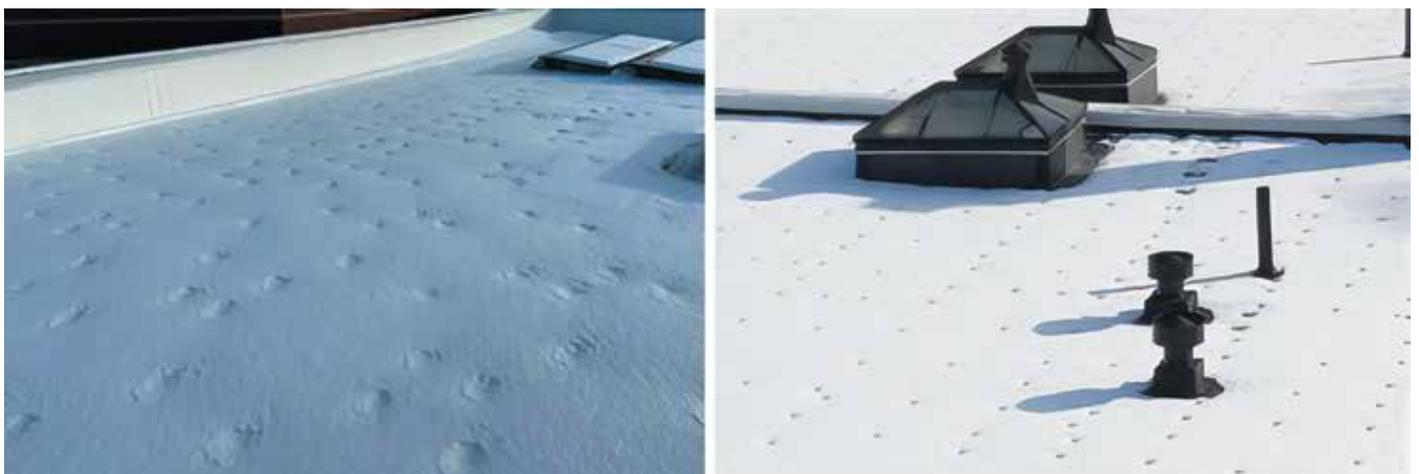
**Figure 1.** Examples of thermal bridging at fasteners on snow-covered roofs.
