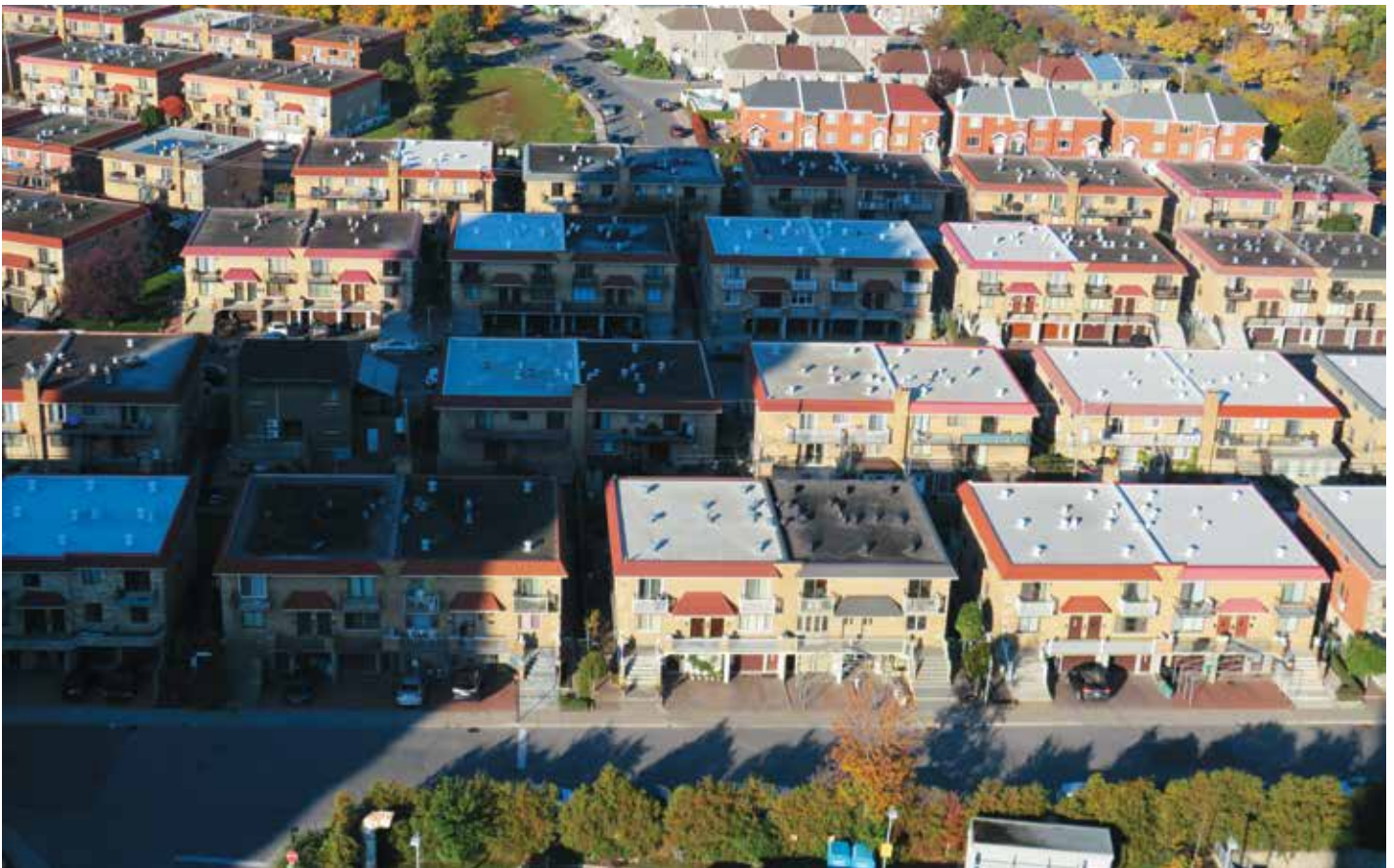
Figure 3. Various roof ventilation strategies employed for similar roofs in the Ahuntsic-Cartierville borough of Montreal.
