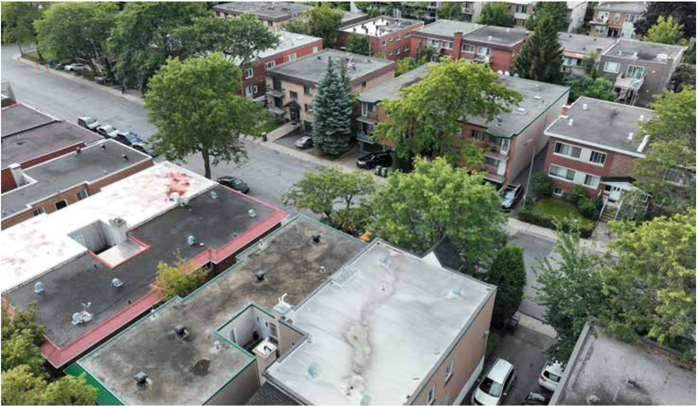
Figure 2. Various roof ventilation strategies are employed for similar roofs in the Notre-Dame-de-Grace borough of Montreal.
