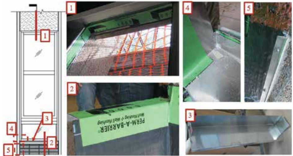
Figure 5. Perimeter waterproofing detailing. (1) Install perimeter waterproofing flashing membrane; (2) Lap sill waterproofing flashing membrane onto cavity wall waterproofing membrane; (3) Form sill pan flashing with fully soldered upturned end dams; (4) Lap jamb waterproofing flashing membrane into sill pan flashing; (5) Install termination bar along the edge of the wall waterproofing membrane.
