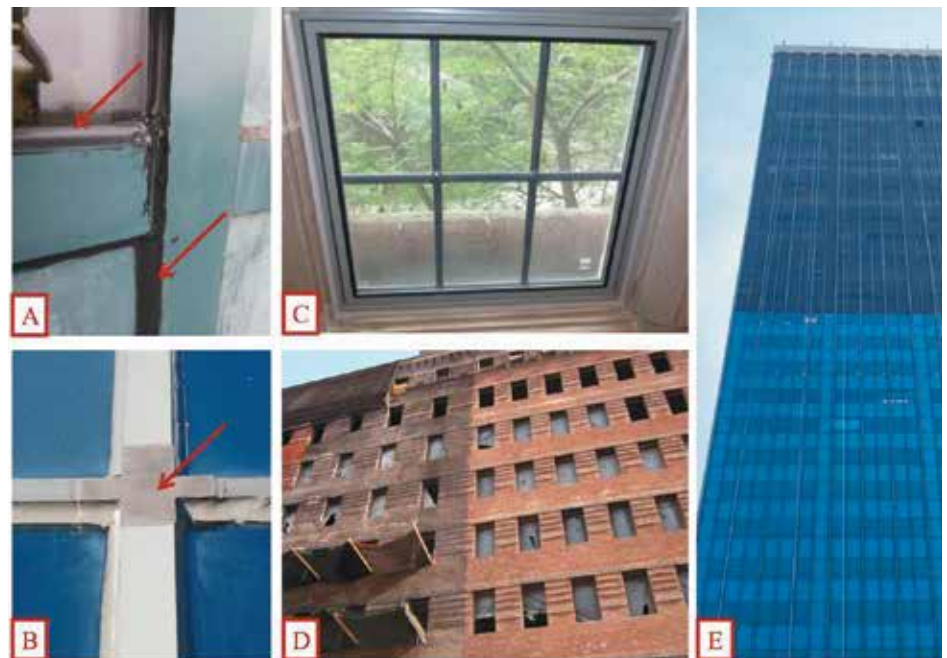
Figure 2. Design options for remediating fenestration issues. (A) New sealant joints; (B) Silicone sheet patches; (C) Storm window installation; (D) Window replacement; (E) Overcladding with curtainwall system.
