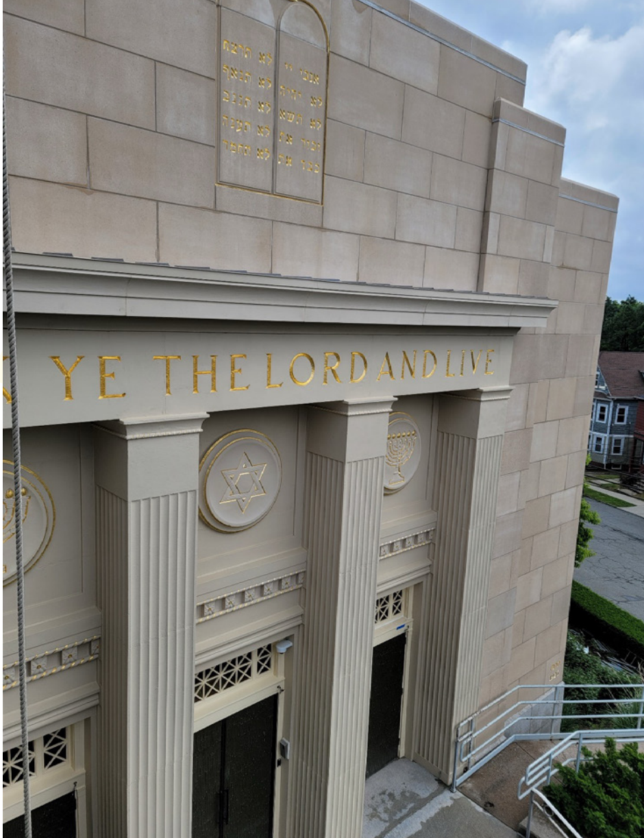
FIGURE 8. The restored Temple Emanu-El with new cast stone units, a glass-fiber-reinforced polymer cornice, and gilding completed.
