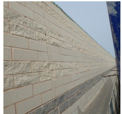
FIGURE 8. Installation of new masonry units during the re-clad construction work.
