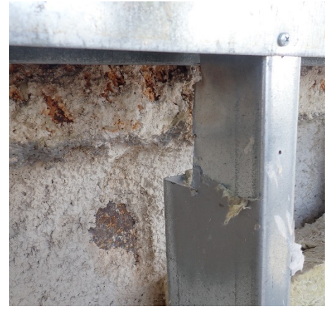
FIGURE 6. Example of photo documentation of backup wall post-sheathing demolition.
