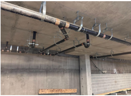
FIGURE 4. Penetrations through the wall of a parking structure that must be sealed airtight to complete the building's continuous air barrier.
