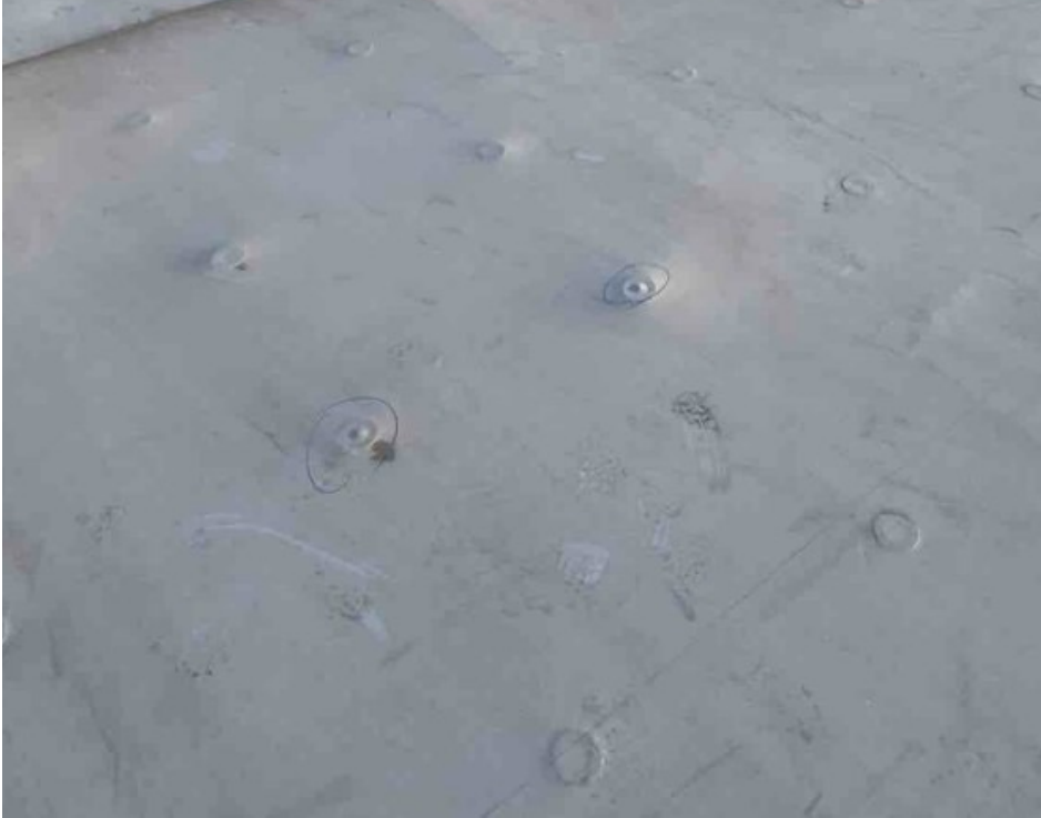
FIGURE 1. Extensive fastener withdrawal with no corresponding wind event.
