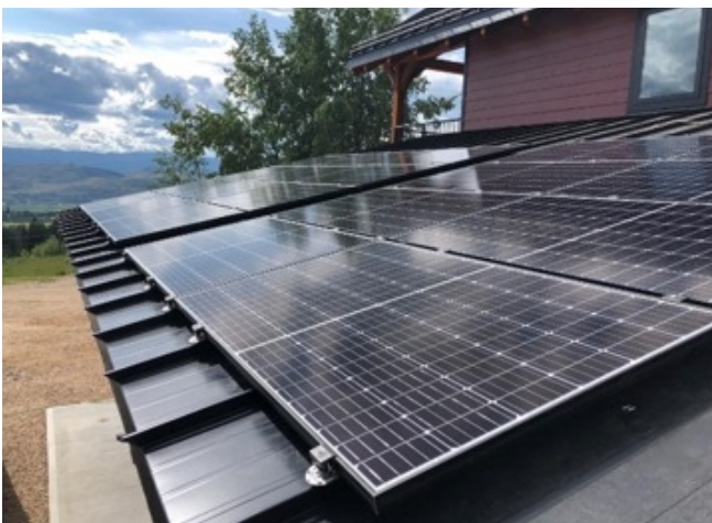
FIGURE 5. Flush Rail-less Mount.
