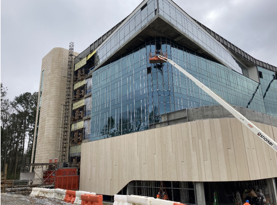
FIGURE 1. Modern building enclosures incorporate many different materials for the exterior walls, fenestration, roofing, and waterproofing system.
