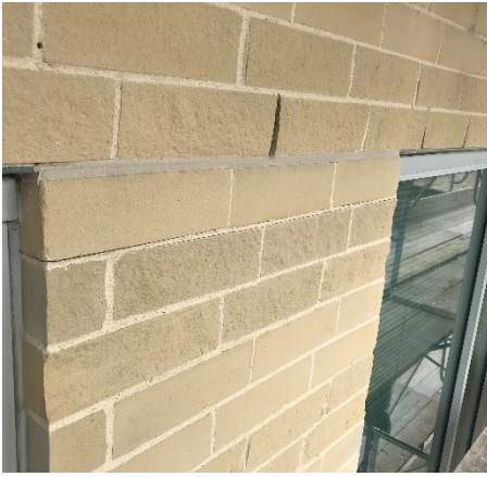
FIGURE 4. Example of photo documentation of masonry condition pre-masonry demolition .
