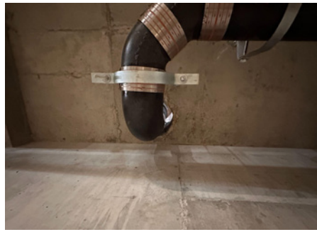
FIGURE 4. Penetrations through the wall of a parking structure that must be sealed airtight to complete the building's continuous air barrier.
