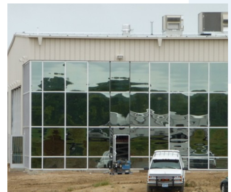
FIGURE 2. Example of roll wave pattern in heat-treated architectural glass.
