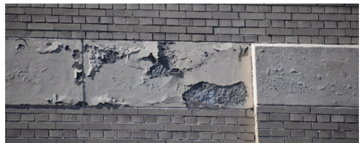
FIGURE 4. Cast stone units at the belt course with blistered and peeling coatings and efflorescence. The top and bottom photos are from 2015 and 2019, respectively. Source: Wiss, Janney, Elstner Associates Inc.
