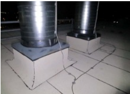
FIGURE 5. Mechanical system ductwork (a) and an FLIR image (b) of the same condition showing the high level of air leakage where the ductwork meets the roof assembly.
