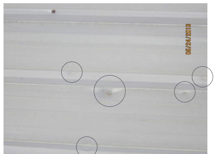
FIGURE 10. Photograph of the dents in the case study roof caused by the Mayfest Storm.
