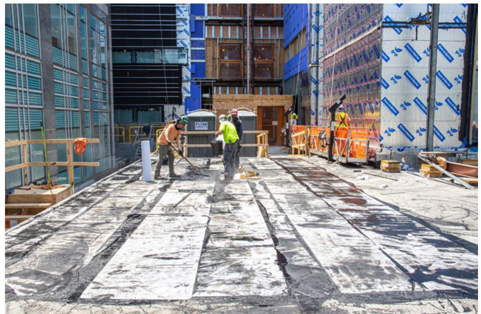
FIGURE 5. HRA Installation in Progress – Credit Jensen Ying.
