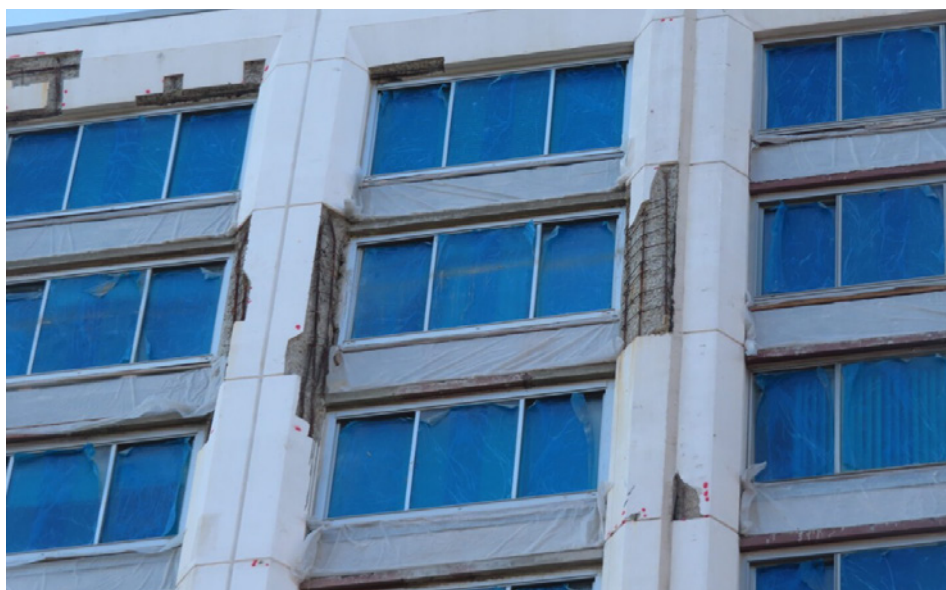
FIGURE 11. In-Progress Concrete Exterior Wall Repairs.
