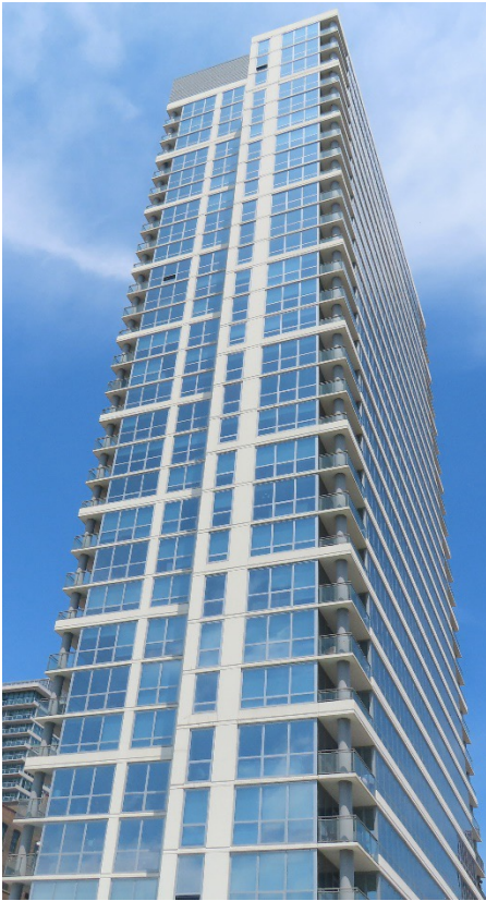
FIGURE 3. Modern Building (Circa 2018) with Exposed Concrete Beams, Wall Areas, Columns, Slab Edges, and Balconies.
