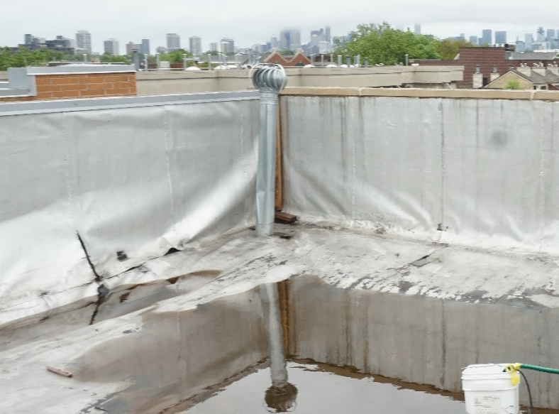
FIGURE 5. Turbine-style roof vent.
