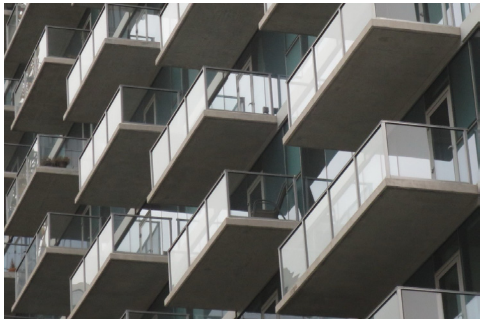
FIGURE 4. Concrete-Frame Balconies Cantilever Beyond the Building Exterior Wall.
