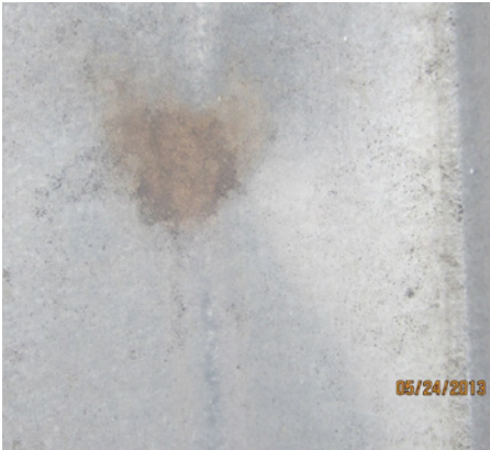
FIGURE 11. Photograph of typical hail-caused indentations with stains in the dents.
