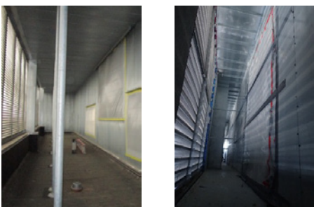
FIGURE 6. Two different plenum shafts where the interior wall must be sealed as part of the air control layer.
