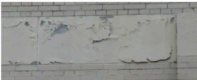
FIGURE 4. Cast stone units at the belt course with blistered and peeling coatings and efflorescence. The top and bottom photos are from 2015 and 2019, respectively. Source: Wiss, Janney, Elstner Associates Inc.
