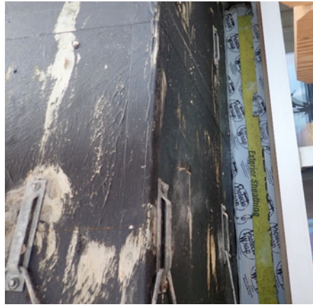
FIGURE 5. Example of photo documentation of masonry cavity wall post-masonry demolition.
