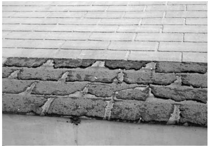
Figure 18: Asphalt shingle showing coated and uncoated sections.
