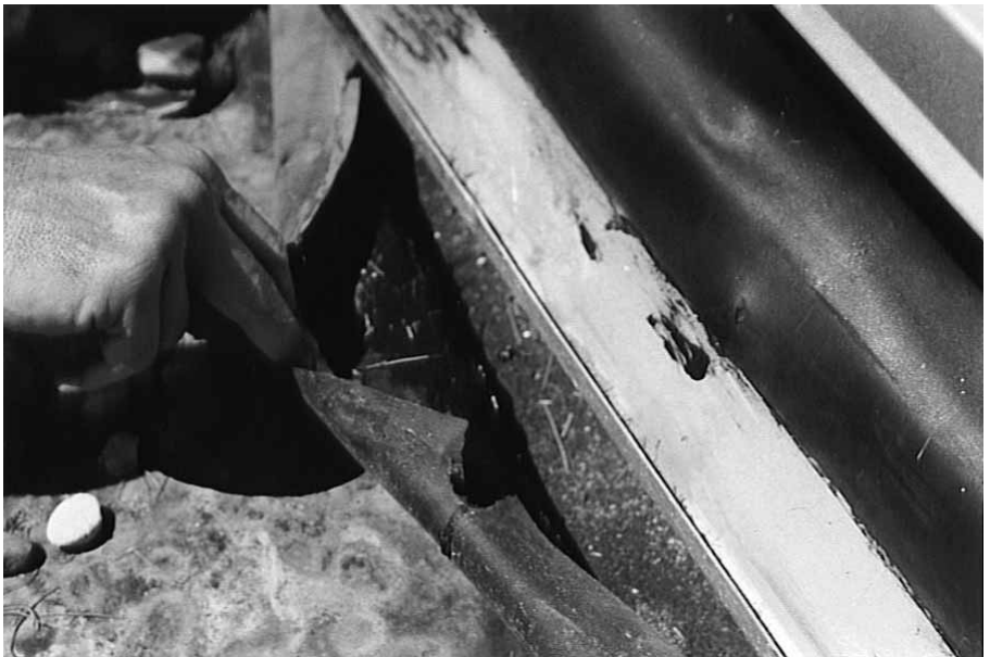
Photo 14: Tear at termination due to membrane shrinkage.
