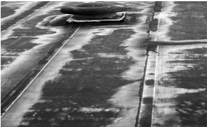
Photo 5: Alligator cracking of aged flood coat of built-up roof.
