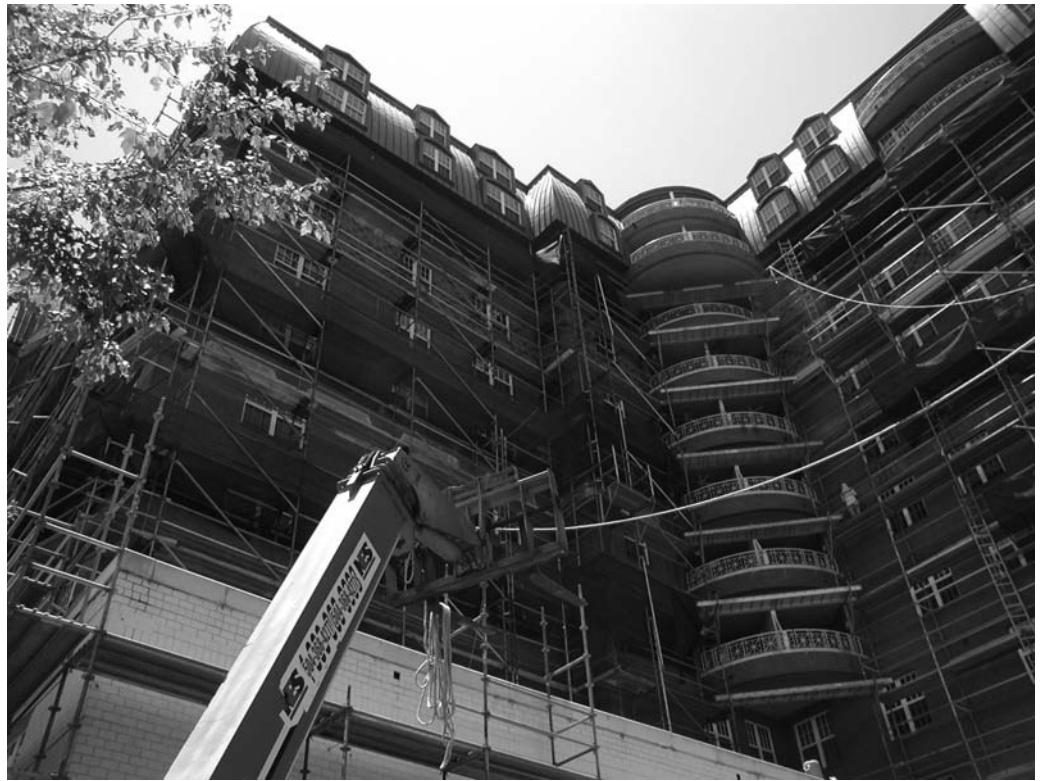
Figure 24 - Extent of scaffolding during renovation for occupied building.
