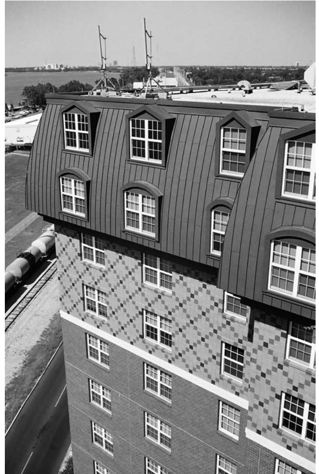
Figure 1 – Typical elevation showing intricate masonry.
