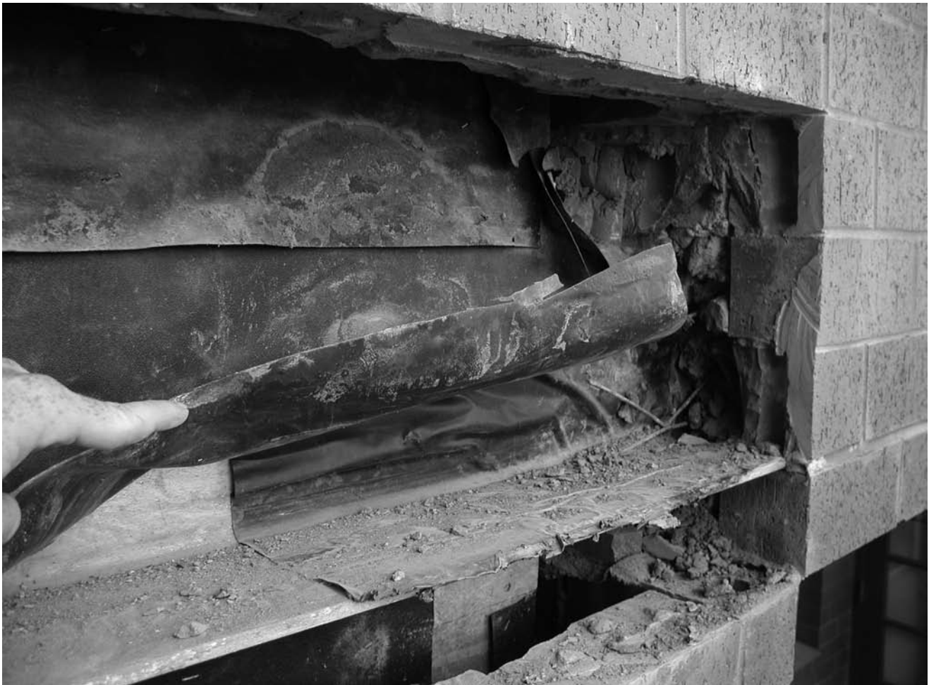
Figure 16 – PVC flashing lap set “dry.”
