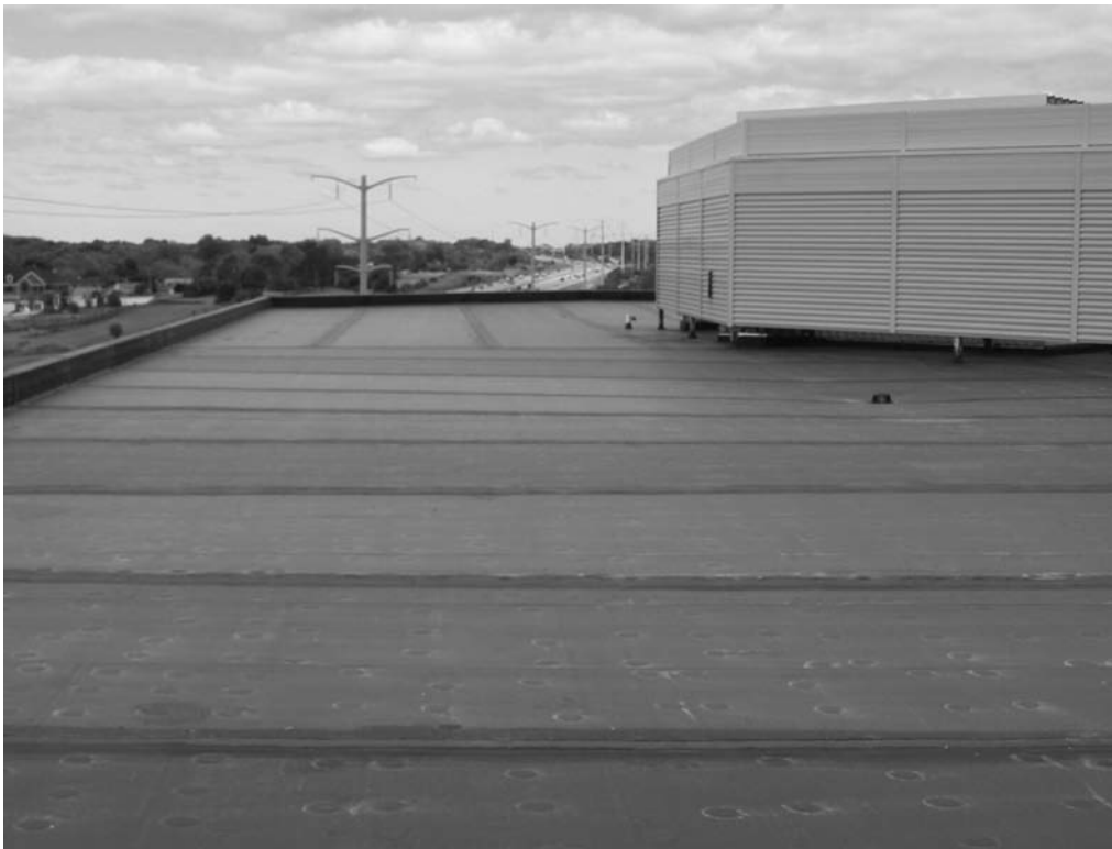
Photo 3 – Illinois Department of Transportation District I building; R-38, 30-year warranty.
