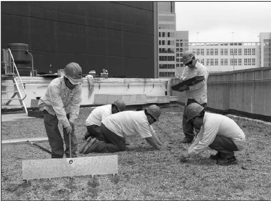
Figure 4 – Vegetation being planted as plugs.
