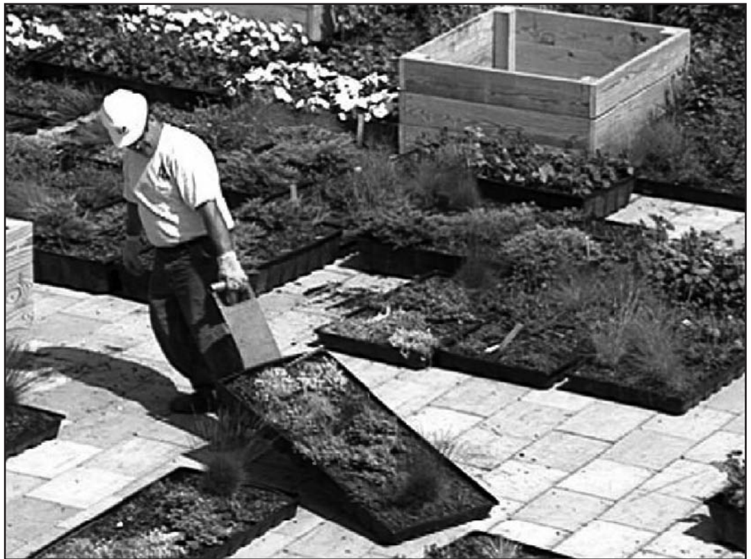
Figure 6 – Example of tray system being installed.
