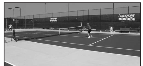
Photo 2 – The author designed this rooftop tennis court on the Lakeshore Athletic Club roof to serve a function besides just watertightness.
