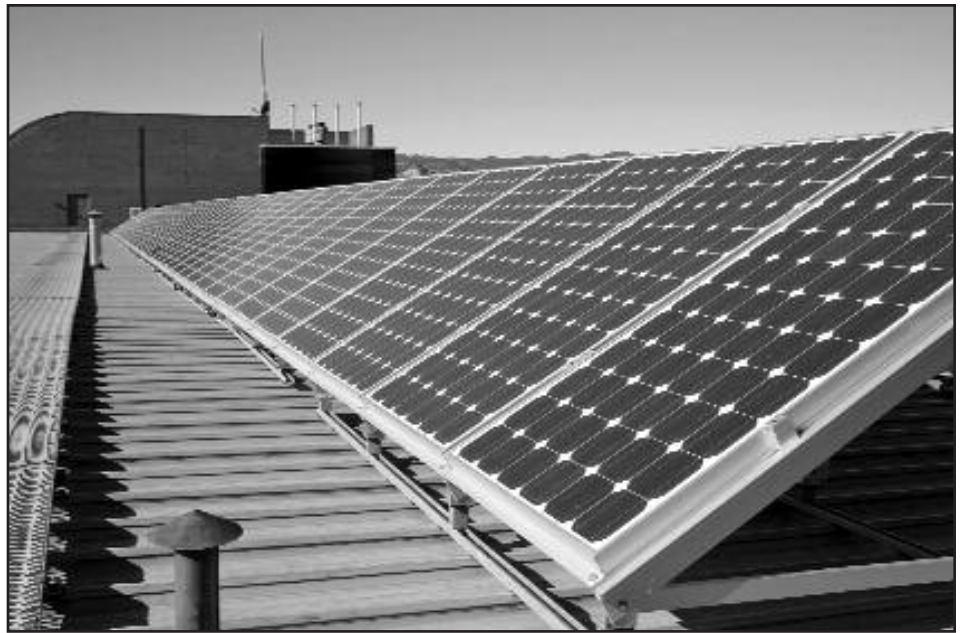
Figure 8 — Panel mounting on standing seam metal roof.
