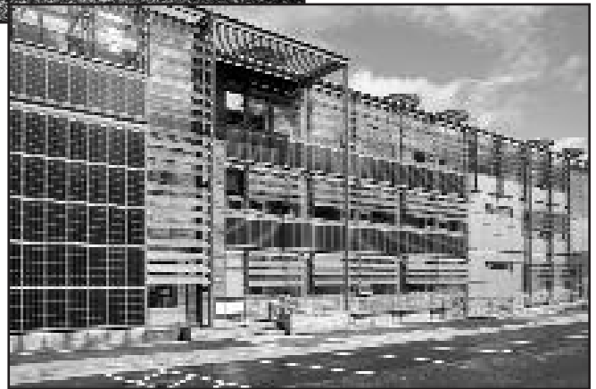
Figure 11 — Building integrated PV (BIPV) in a curtain wall.
