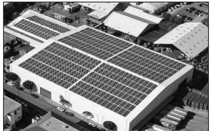
Figure 4 – Flexible thin film on a large roof.
