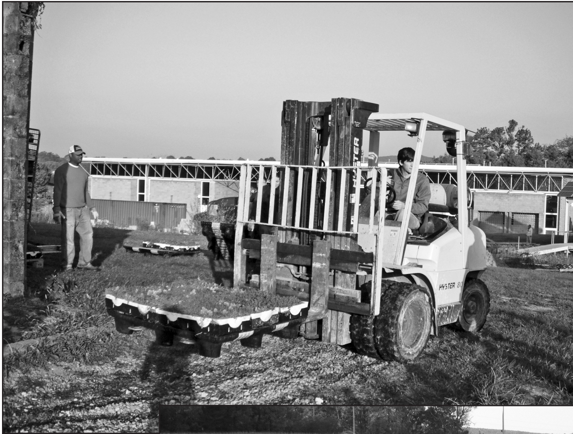
Figure 3 – Modules brought to platforms via forklift.
