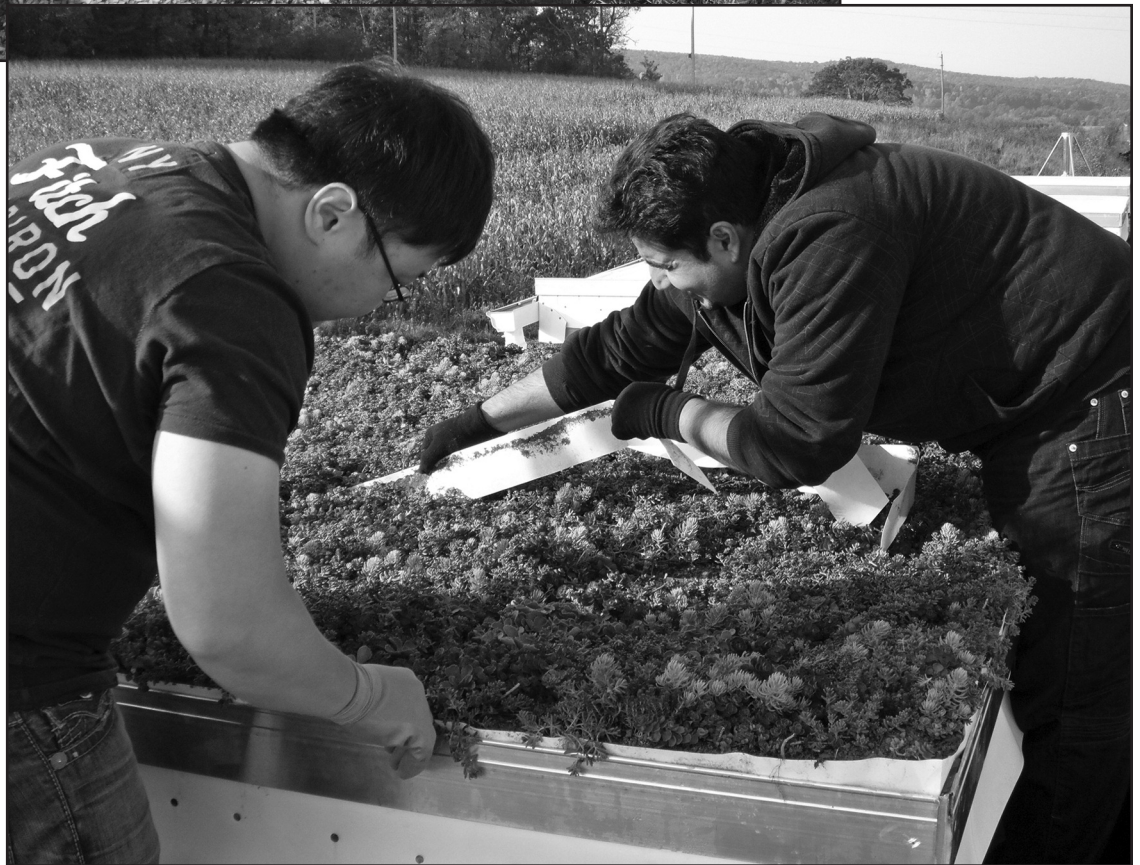
Figure 4 – Student volunteers installing prevegetated modules.
