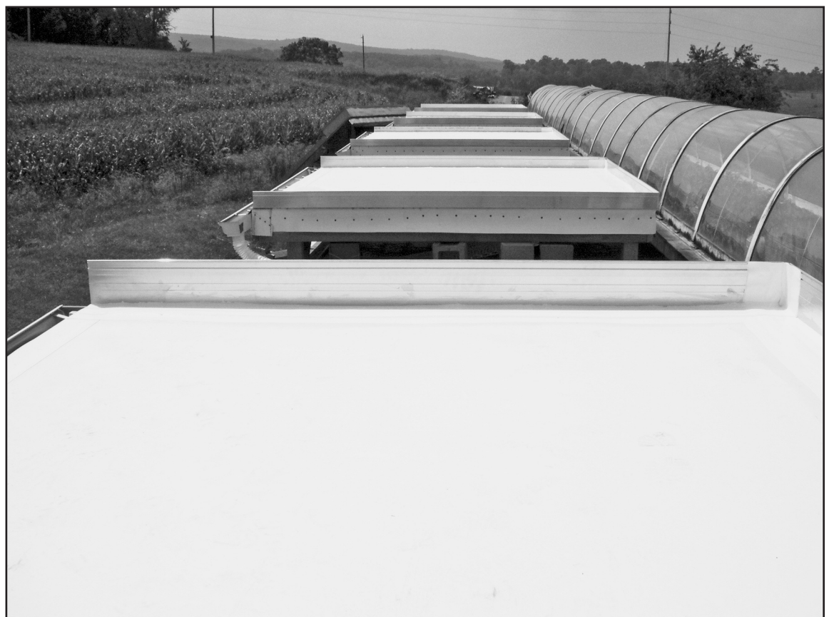
Figure 2 - Waterproofed platforms awaiting vegetated module installation.
