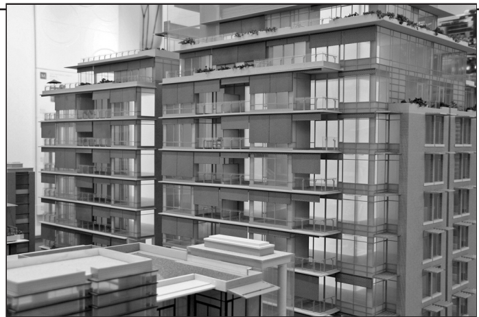
Figure 3 - Shading strategy: automated vertical shades on the west façade (left), and horizontal shades on the southern elevation (right).
