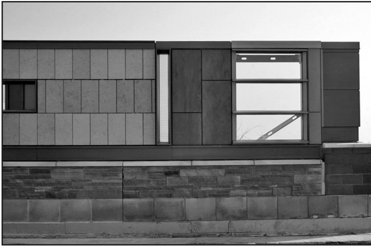
Figure 7 – Site visual and assembly mock-up with various materials used in the building wall.
