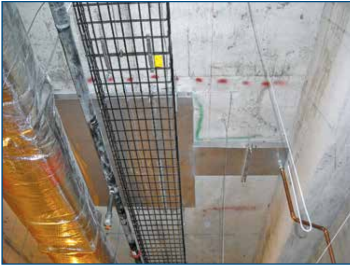
Figure 8 – Drain pan system.
