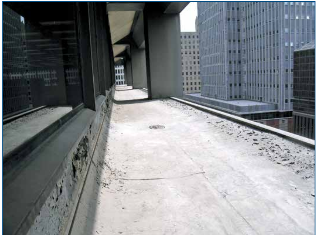
Figure 9 – Typical balcony, original condition.
