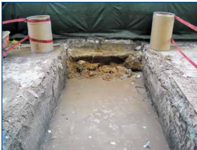
Figure 4 – Concrete “catch basins” at street.
