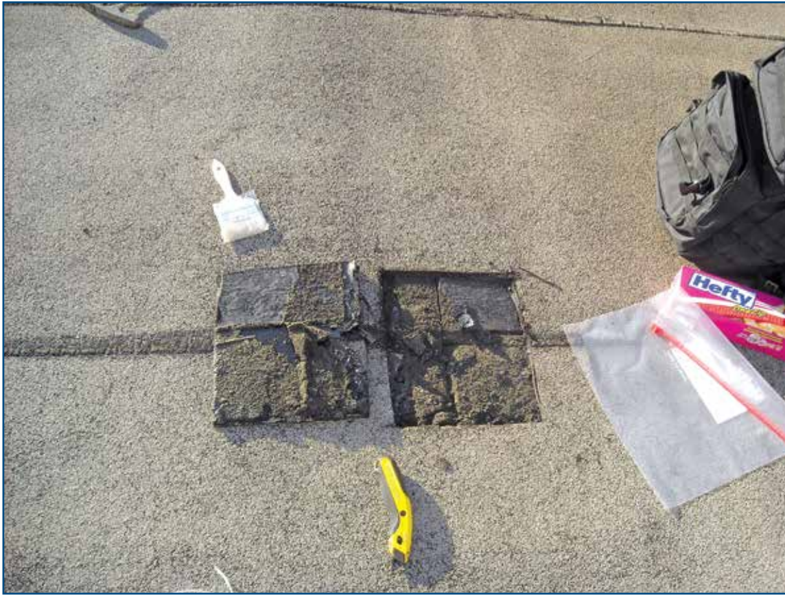
Figure 12 – Roof test cuts.
