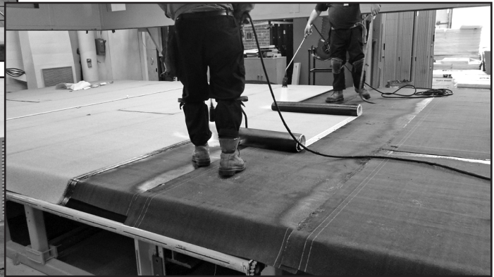
Figure 5D – Cap sheets were torched to the base sheet layer.
