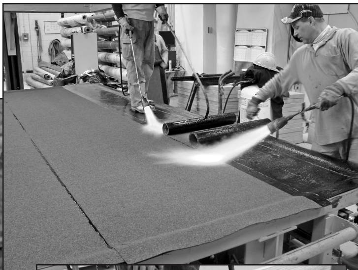
Figure 4D - Cap sheets were torched to the base sheet layer.
