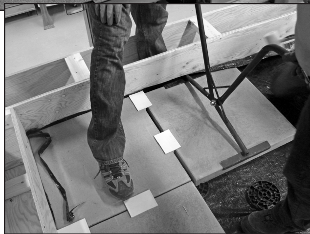
Figure 4F - 2-in. x 2-ft. x 2-ft. (51-mm x 1219-mm x 1219-mm) concrete pavers were placed on the top of the woven polyethylene fabric with paver supports 6 in. (152 mm) in diameter and 3/4 in. (19 mm) thick.
