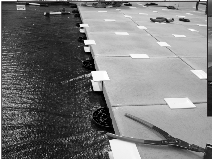
Figure 4G - Pavers were interconnected with 5-in. x 3 3/4-in. x 2 1/2-in. (127-mm x 83-mm x 64-mm) plastic H clips.
