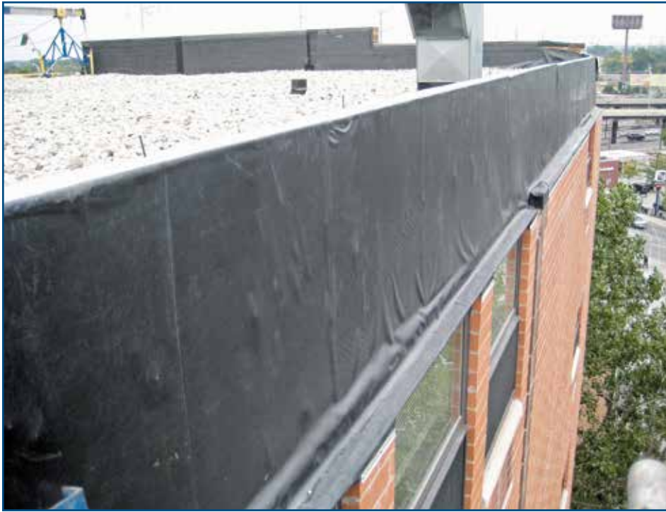
Figure 11 – Temporary treated wood-framed parapet wall installed in 2008.
