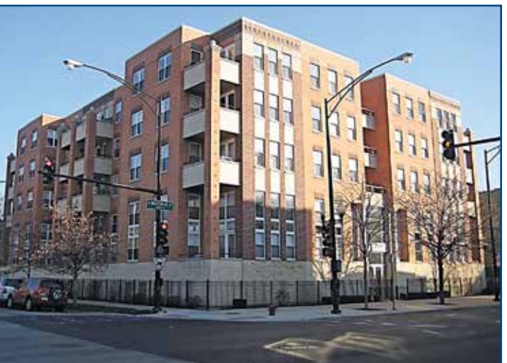
Figure 5 – Building façade after completed repairs.
