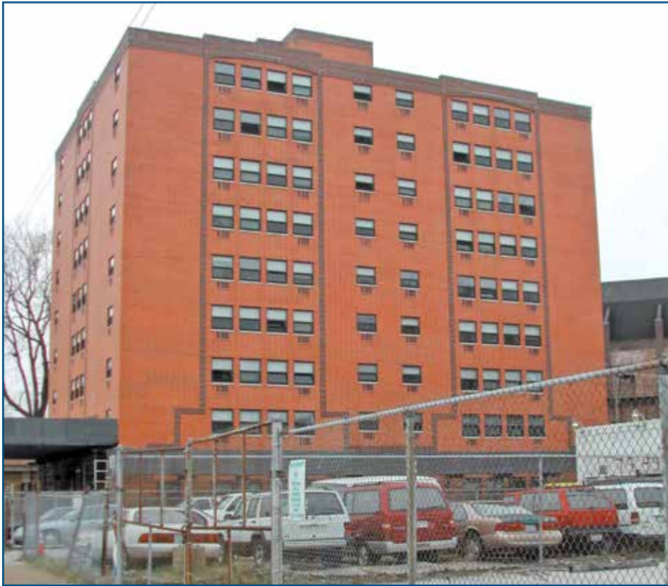
Figure 6 – View of the south façade of the building in 2007.
