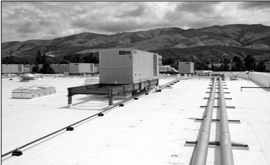
Figure 17 – Well-drained reflective roof.
