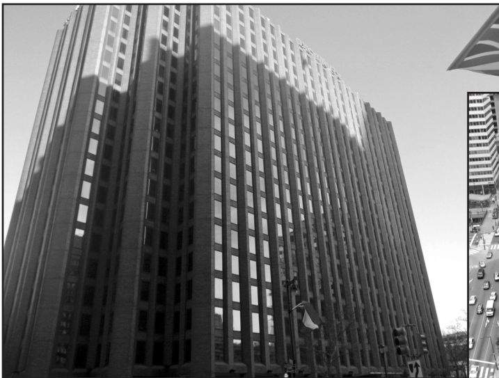
Photo 1 – Typical façade overview of subject building.
