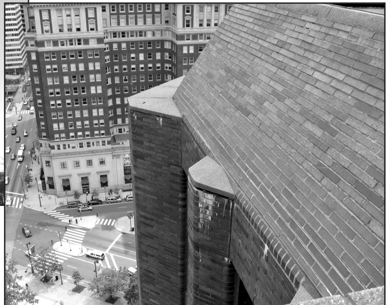
Photo 2 – Top of mechanical chase projections and sloped wall.
