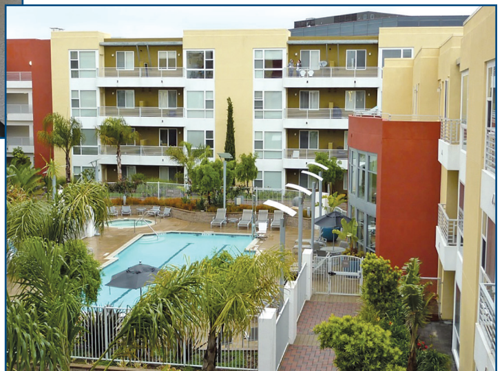
Figure 7 – Typical podium with concrete topping and pavers, shade structures, fences, planters, trees, pool, spa, light pole, free-standing walls, etc. integrated with building walls, fences, doors, pools, and planters.
