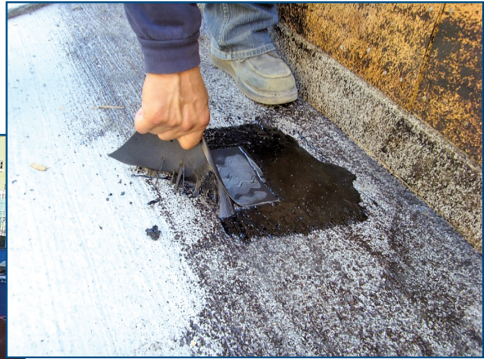
Figure 11 – Adhesion of membrane with sheet neoprene.
