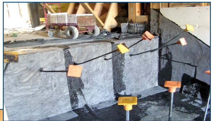
Figure 14 – Waterproofing around reinforcing steel.
