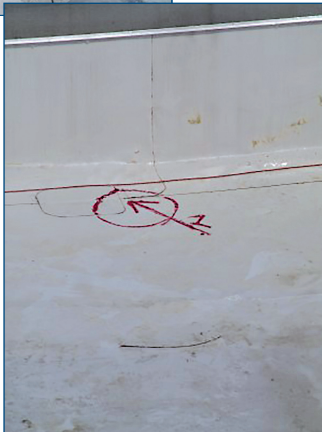
Figure 20 - Using potentiometer to discover source of leaks.
