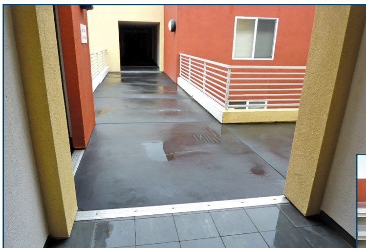
Figure 6 – Elevated public walking surfaces on wood deck with colored concrete and porcelain tile wearing surfaces, integrated with handrails, doors, exterior walls, elevators, etc.
