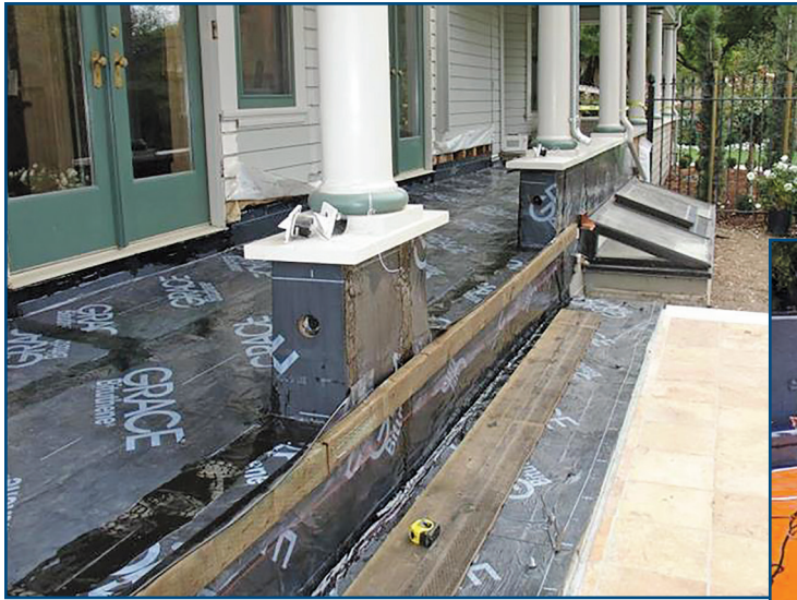
Figure 8 – Combination self-adhered modified-bitumen membrane with fluid-applied waterproofing.
