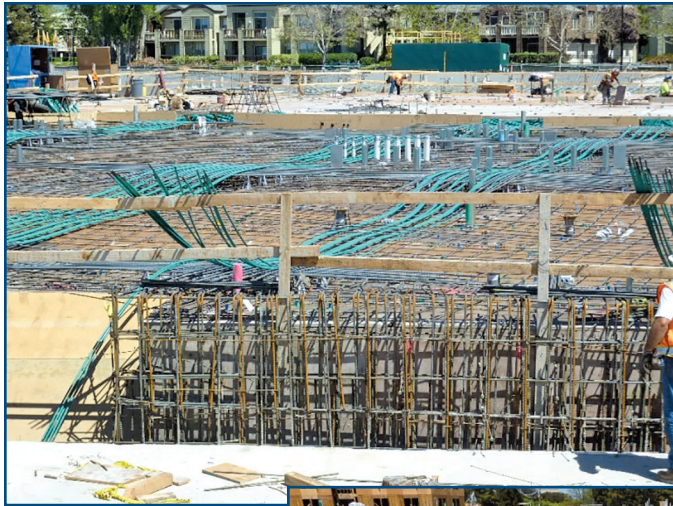
Figure 3 – Podium slab with tensioning cables and reinforcing steel.
