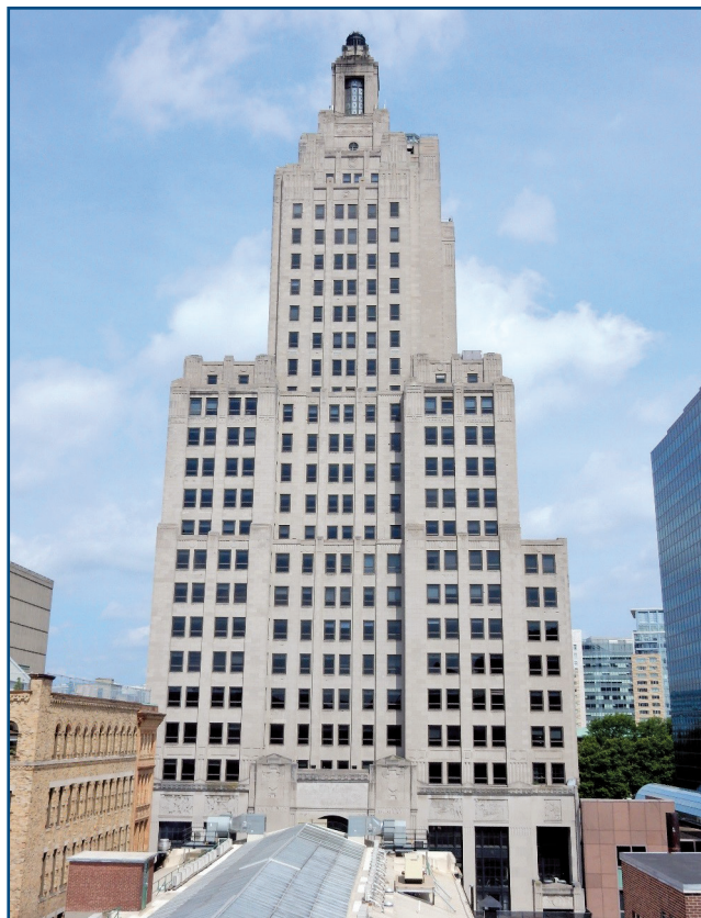
Figure 1 – Building where rope access techniques were used in lieu of a swing stage.
