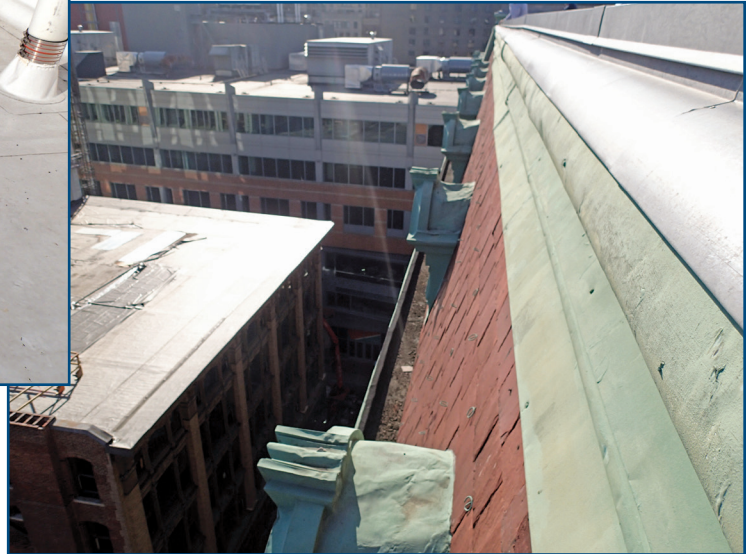
Figure 8 – Steep-sloped mansard roof areas of educational building in Figure 5.
