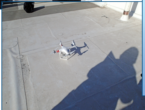
Figure 10 – Drone ready to take off from low-sloped roof area.
