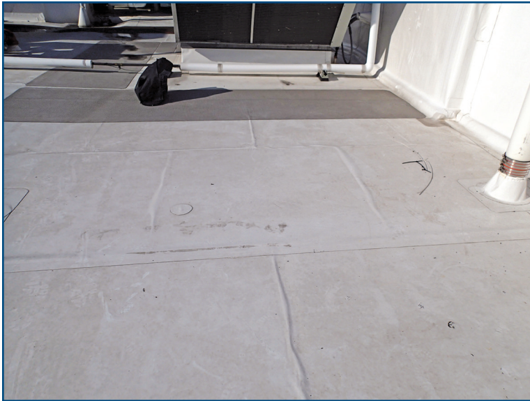
Figure 7 – Low-sloped roof areas of educational building in Figure 5.
