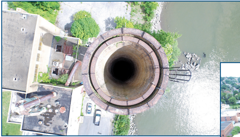
Figure 16 – Image from a drone, looking straight down a chimney.
