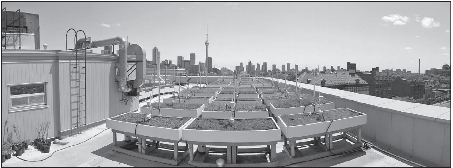
Figure 1 - View of the GRIT Lab research facility showing all 33 green roof bed modules.
