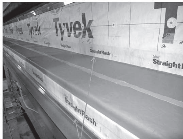
Self-adhered flashing under horizontal Z-girts.
