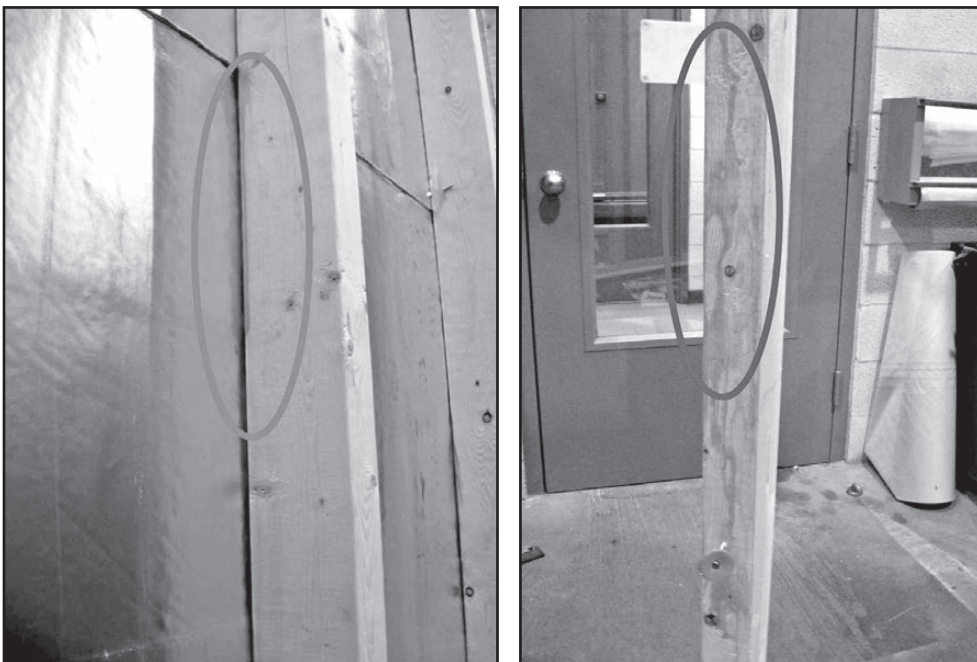
Figure 10 – Water intrusion at foam sheathing joints following laboratory wall assembly testing per ASTM E2357 integrated with thermal cycling.
