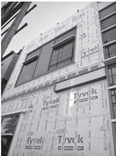
Self-adhered flashing under brick ties.
