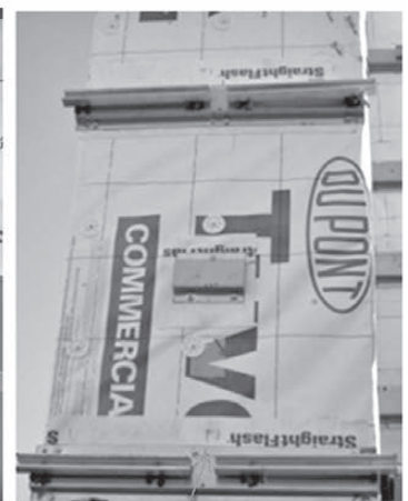
Self-adhered flashing under metal hat channels.
