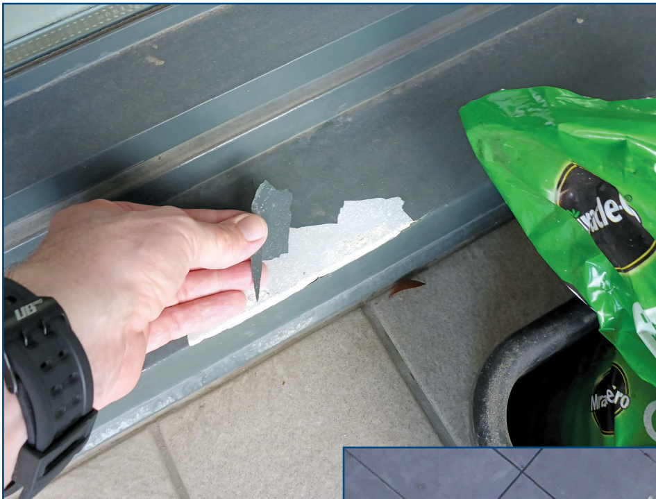
Figure 12 – Example of paint failure.
