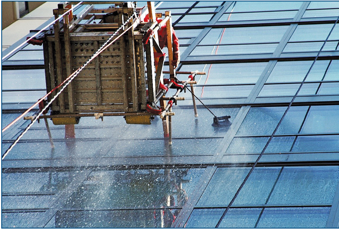
Figure 2 – ASTM E1105 water testing of a curtainwall.
