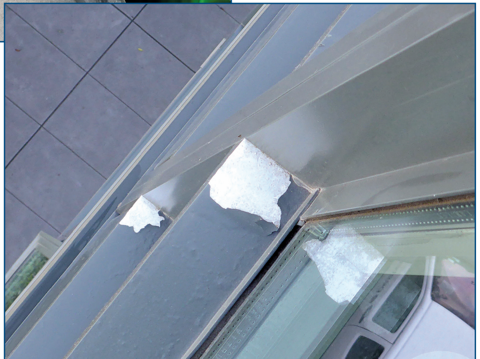
Figure 13 – Example of paint failure.
