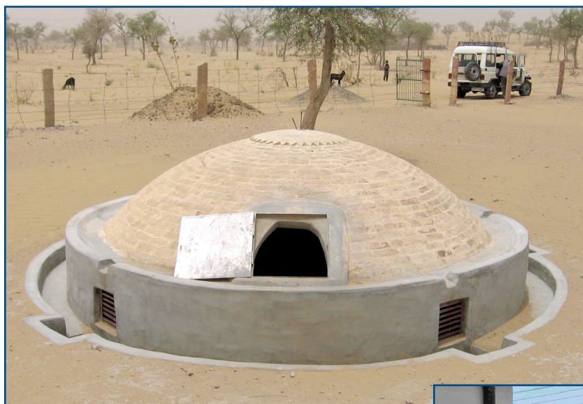
Figure 2 – Tanka, a traditional Indian roof water catchment system. Source: P.C. Chatterji. “Status of Ground Water in Rajasthan.” Institute of Dev. Studies, Volume I, pp. 96 (1993).
