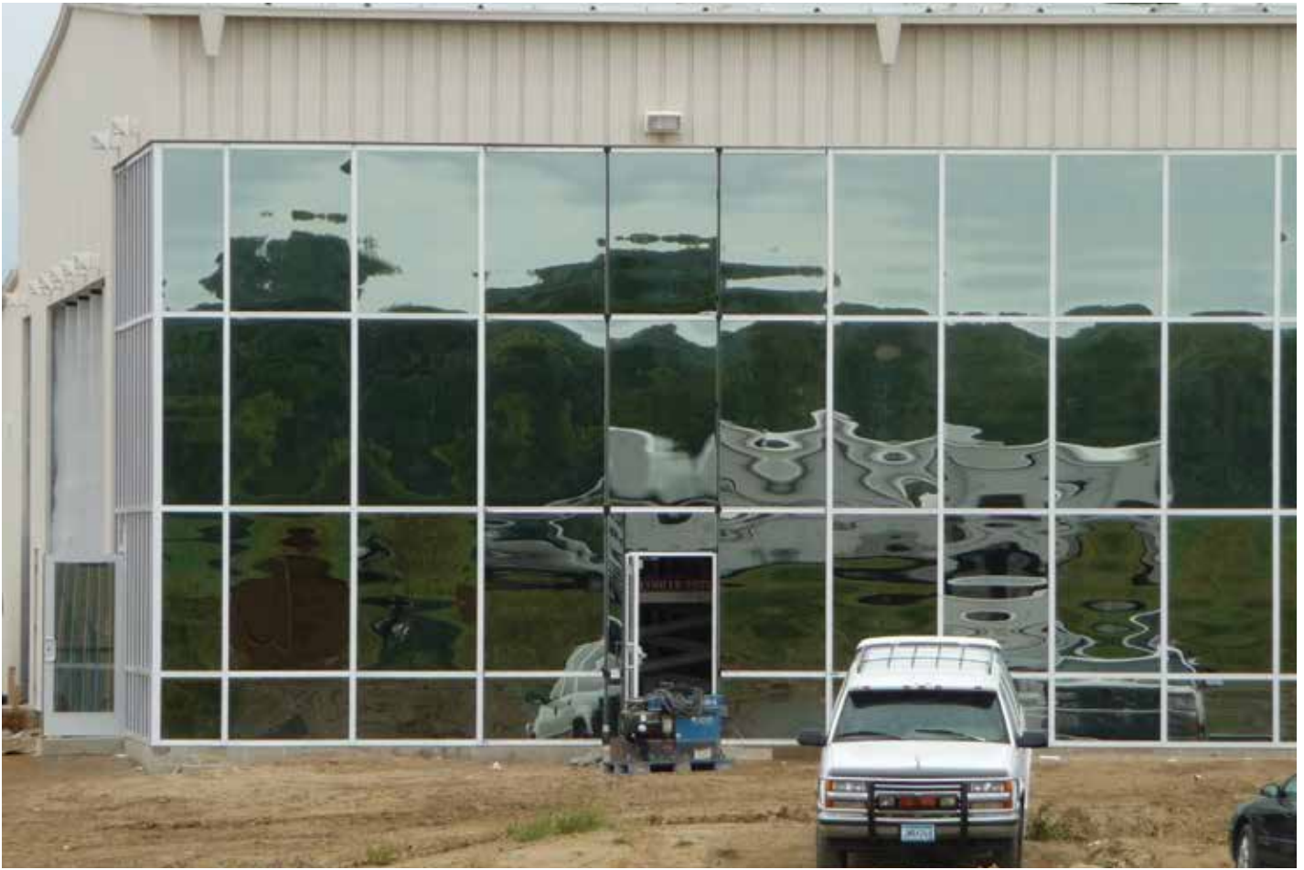
Figure 2. Example of roll wave pattern in heat-treated architectural glass.
