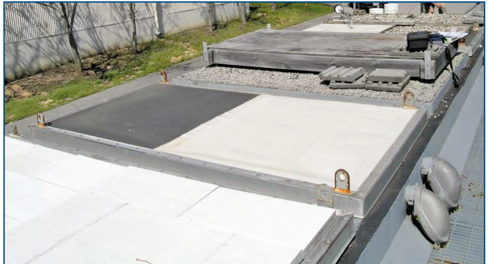
Figure 1 – Test roof sections on the Roof Thermal Research Apparatus.
