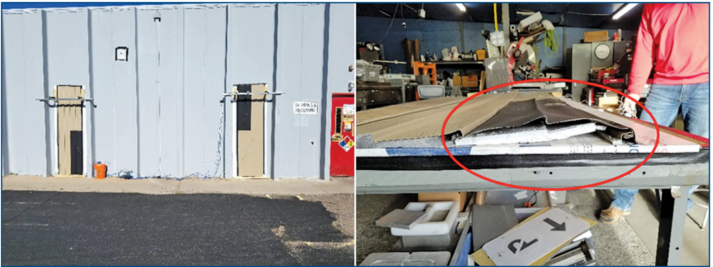
Figure 7 – Initial experiment setup (left); delamination and warping of siding (right).
