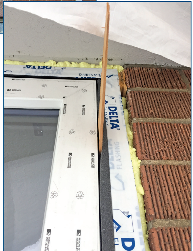
Figure 7 – Passive House window and balcony door installation in an existing building.
