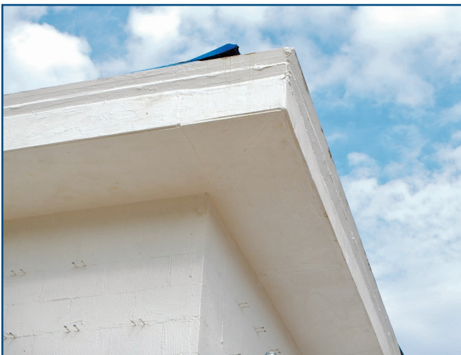
Figure 16 – Fire Station A. Closeup view of the liquid-applied air barrier creating airtight assembly at the roof soffit.
