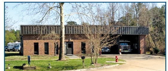
Figure 1 - The original fire station before demolition and construction of the new fire station.
