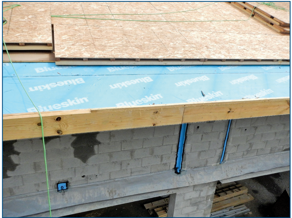
Figure 24 – Fire Station B. View of installed vapor/air barrier on the roof deck prior to installation of the compact ventilated roof system insulation and roof sheathing.
