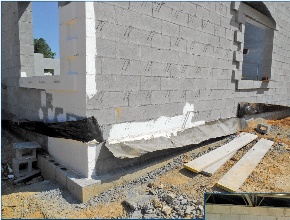
Figure 14 – Fire Station A. View of ongoing preparation work of the liquid-applied air barrier above and below the through-wall flashing tying it into the foundation wall, rough openings, and through-wall flashing.
