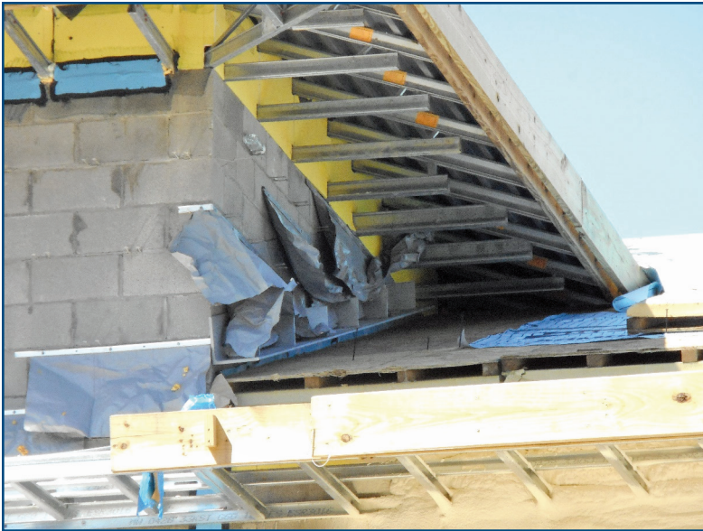
Figure 22 – Fire Station B. Close-up view of soffit where detailing and preparation work for the air barrier system (SPF) is ongoing using transition membrane and sealants.
