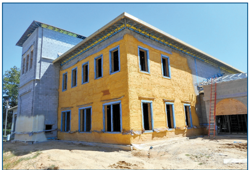
Figure 21 – Fire Station B. View of SPF air barrier over CMU backup wall. Note areas of detailing around windows and other penetrations.
