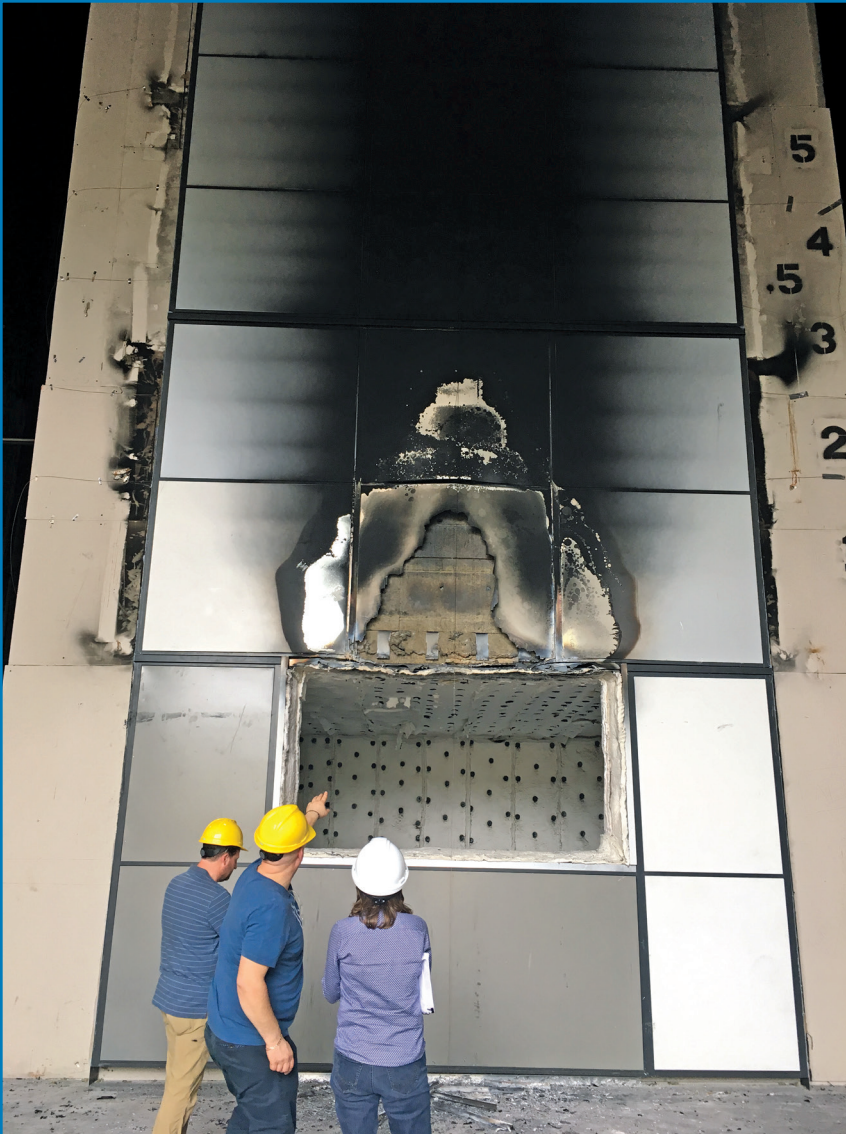
Figure 4 – Apex of burn pattern above window opening.
