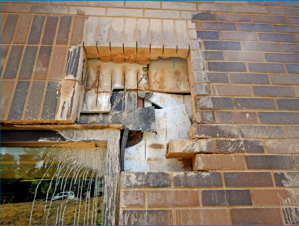
Figure 4 – Inspection location at a window head corner revealing the condition of the loosely placed rigid foam board sheathing and poorly installed PVC flashing.
