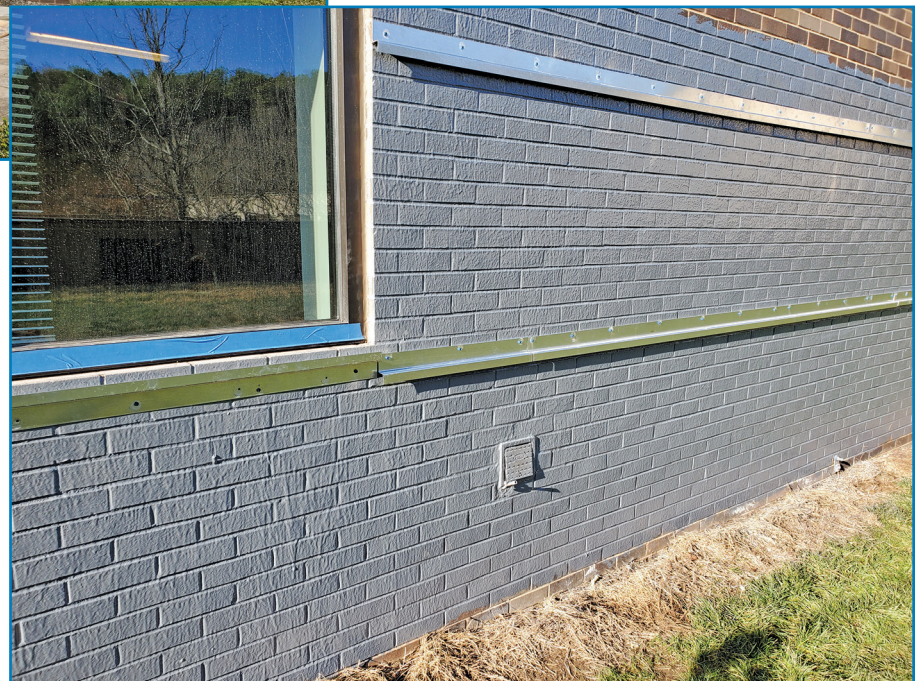
Figures 7 and 8 – Ongoing installation of the liquid-applied vapor-permeable air and weather barrier being applied to exterior gypsum sheathing and brick cladding.
