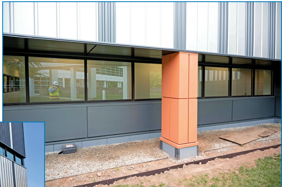
Figure 12 – Finished metal cladding system depicting custom colors and variation of panel types and details.
