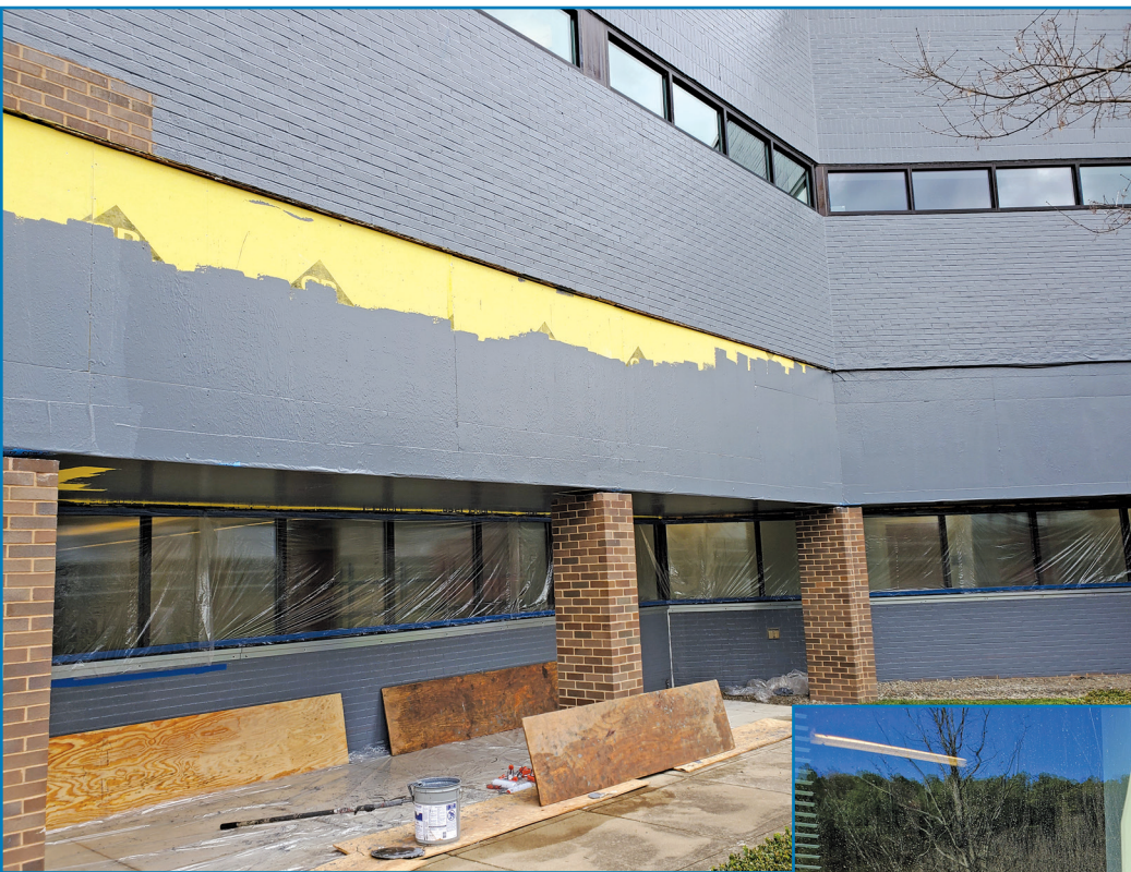
Figures 7 and 8 – Ongoing installation of the liquid-applied vapor-permeable air and weather barrier being applied to exterior gypsum sheathing and brick cladding.
