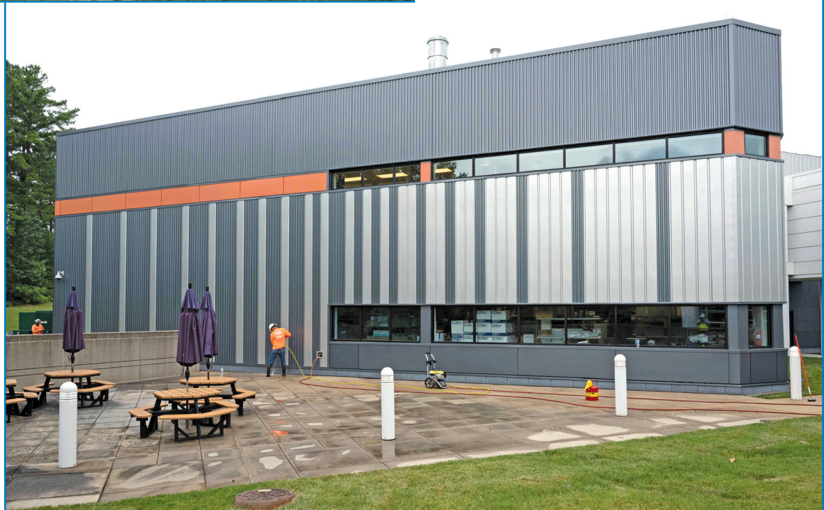
Figure 15 – Another view of the completed end wall with custom colors and variation of metal building wall panels.
