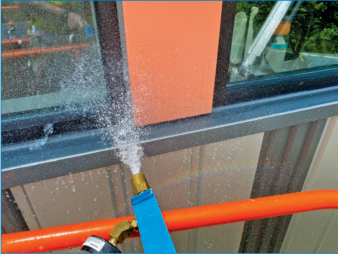
Figure 11 – The installed cladding system was tested using ASTM spray nozzle techniques.
