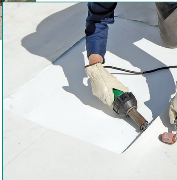
Figure 12 – Repair of aged TPO membrane with a new patch welded to the aged core. Image courtesy of WSRCA.
