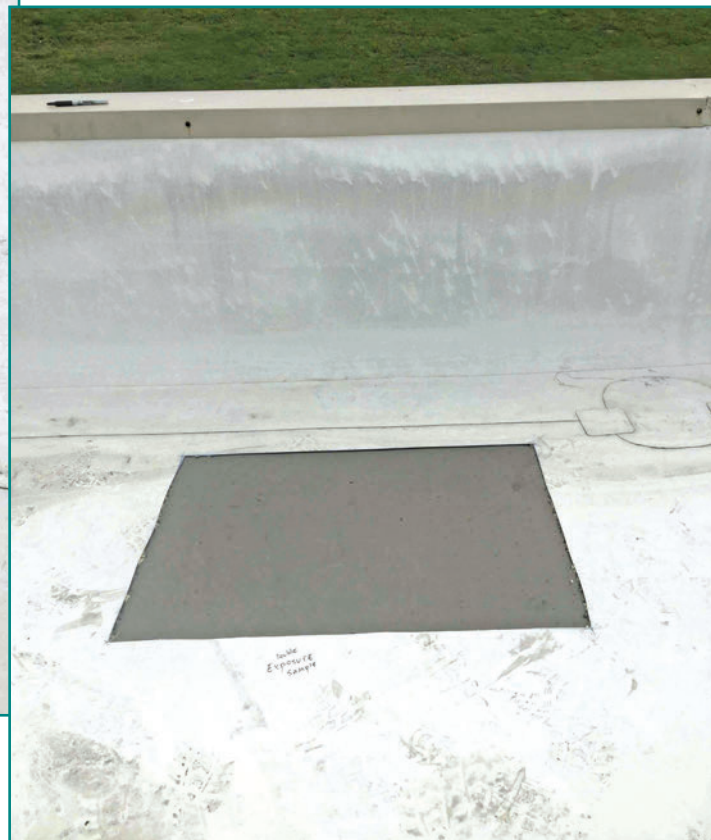
Figure 2 – Typical north parapet, 30 inches in height.
