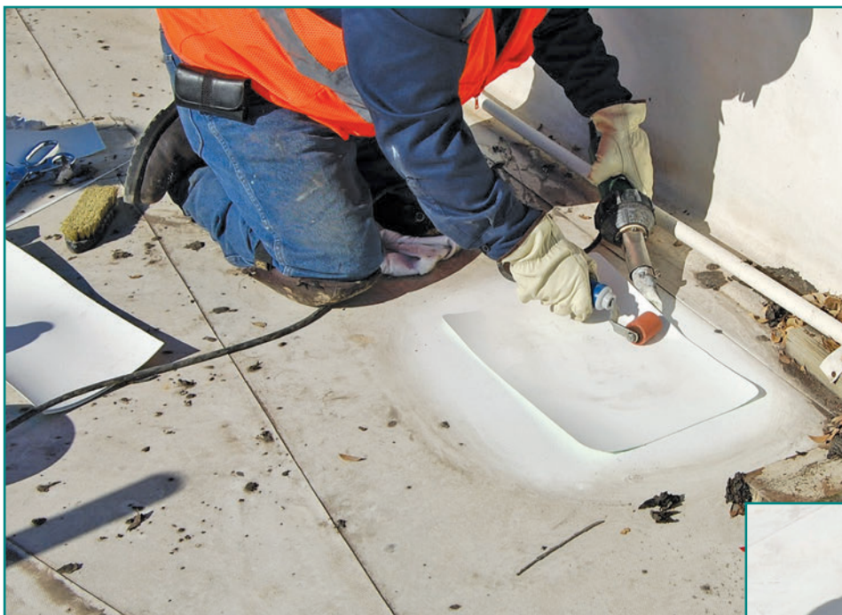
Figure 11 – Repair of aged TPO membrane with a new patch welded to the aged cap. Image courtesy of WSRCA.
