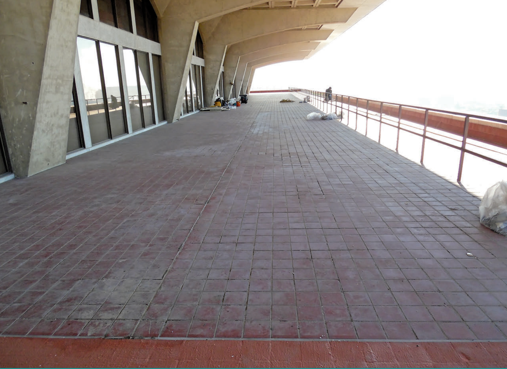
Figure 6 – Case Study 2 ninth-floor terrace with quarry tile pavers.
