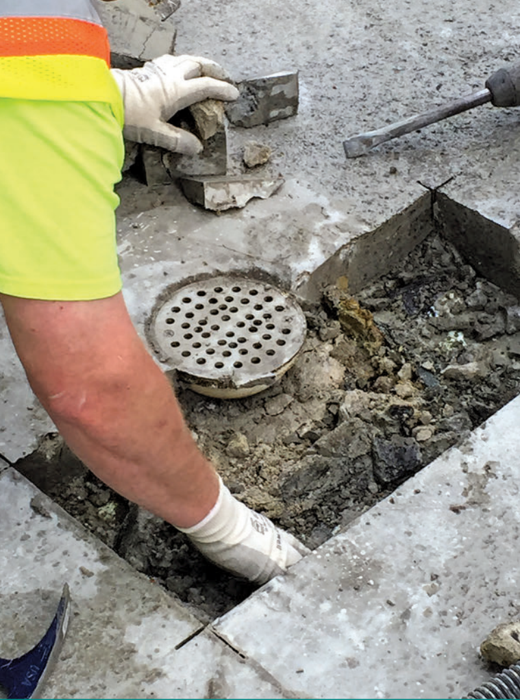
Figure 3 – Exploratory opening at plaza drain.
