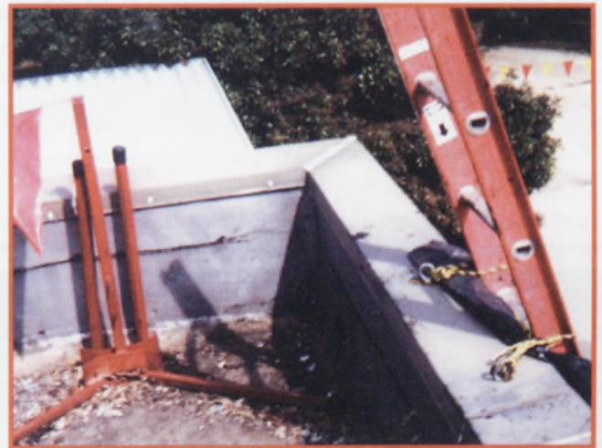
Consultants often use contractors' ladders. This ladder is properly secured and safe to use to access the roof.
