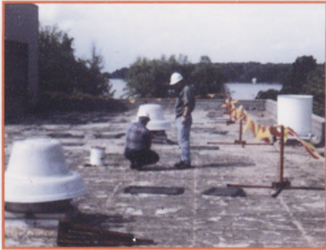
Contractor warning lines also apply to consultants in most cases.
