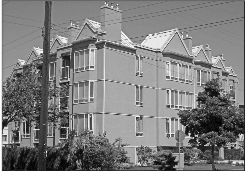
Figure 1 – Building 2 of the monitoring study overview: a typical four-story, low-rise structure with rainscreen walls.
