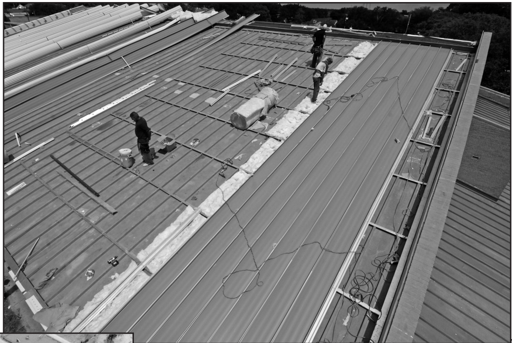
Figure 2 – New metal roof over existing steep-slope metal roof.
