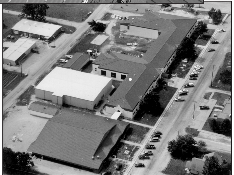
Figure 4 – New metal steep-slope roof after retrofit.
