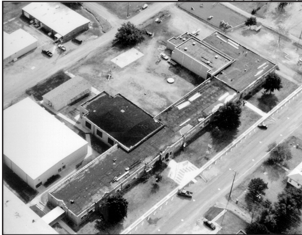
Figure 3 – Existing low-slope roof before retrofit.
