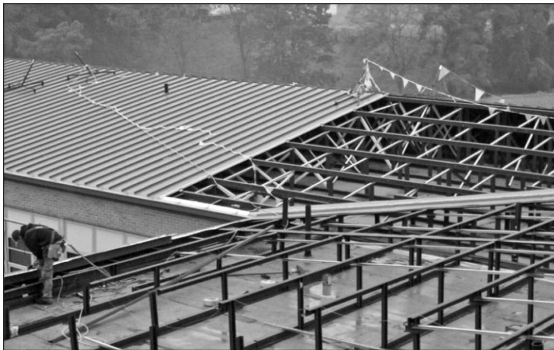
Figure 1 – New steep-slope metal roof over existing low-slope roof.
