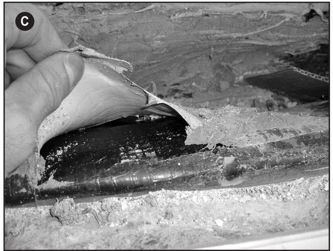
Photo 1A — A seismic expansion joint is located in the reentrant corner of an H-shaped building complex. The joint continues vertically and horizontally along this gridline. Fire resistance and thermal insulation are required, since the joint runs through a living unit. 1B — A polymeric bellows material was used, and corners and transitions were detailed using excessive sealant. 1C — The sealant used does not bond to the bellows material, creating gaps at the bellows joints and transitions.
