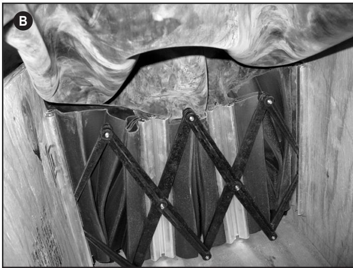
Photo 3A — Mock-up of 14-in seismic expansion joint using preformed joint covers and assembly. Main purpose for the mock-up was to review transition of horizontal bellows with the vertical joint assembly. Notice how the transition is made by carving the roof bellows around the aluminum intermediate frame and sealing them to these frames using sealant material. 3B — Inboard side of the joint cover showing the adjustable frame used to center the joint system in the event of movement. 3C — Joint cover assembly installed on building, showing transition of vertical and horizontal seismic joint. 3D — Joint cover detail provided by manufacturer shows a secondary backup polymeric membrane (as seen in 3A) to function as bellows, which, however, does not provide a tie-in to lap over the WRB for non-face-sealed walls.
