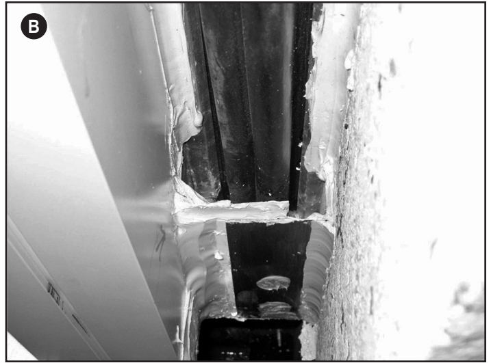
Photo 4A — 2-inch vertical seismic joint between precast concrete panel and curtain wall system. Joint cover system consists of extruded polymeric cover system with integrated bellows attached to aluminum frames (mounting rails). The frames are bedded in sealant on each side and bolted to the adjacent façade systems.; 4B — The interior side of the seismic joint showing the bellows and the frames set in thick beds of sealant. During performance testing, voids in the sealant were discovered, and additional sealant was applied resulting in thick vertical beads of sealant on both sides. The base of the seismic joint consists of a two-piece sheet metal base flashing that is sealed together and onto the wall surface with sealant. Once again, the use of sealant at the base flashing is excessive; and yet, during the first round of testing, the flashing failed.
