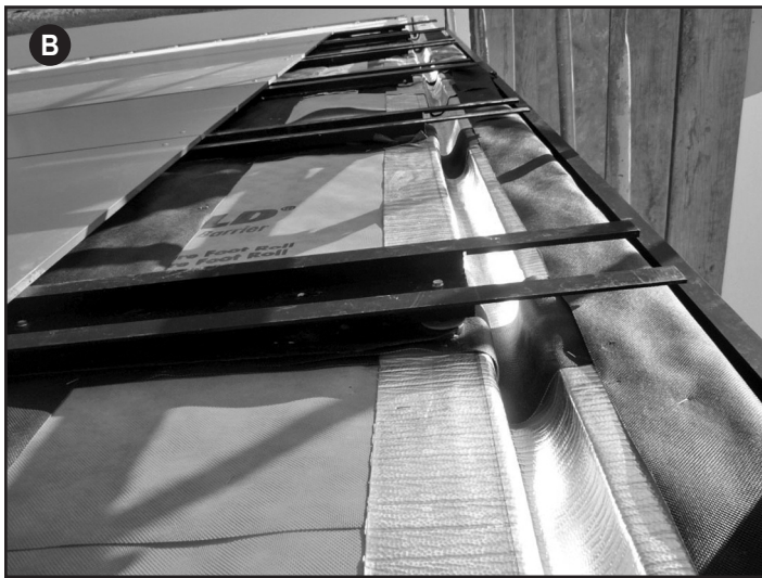
Photo 5A — A 2¼-in vertical seismic joint and 1-in interstory horizontal drift joint intersection. 5B — Vertical sheet membrane bellow, continuous with no mechanical panel attachments within the joint. 5C — Membrane bellows unadhered within drift joint to allow for movement. 5D — Bellows termination is inadequate and will not be able to take any movement, resulting in damage to the membrane bellows.
