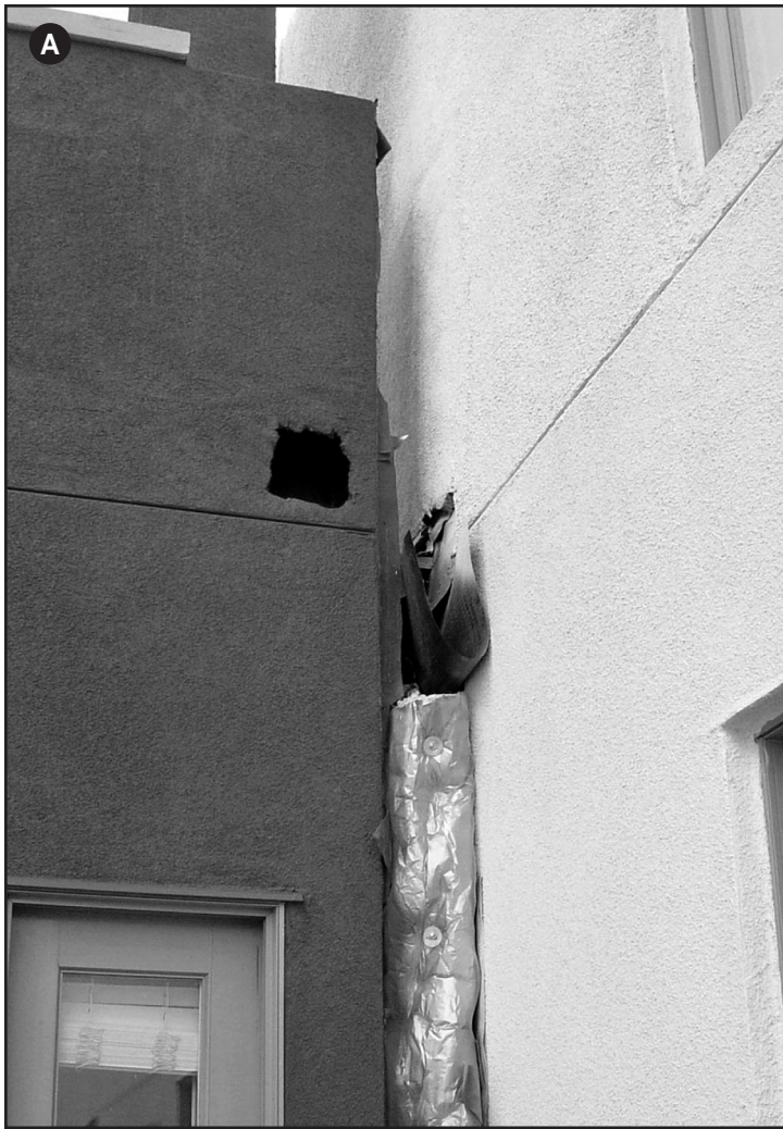
Photo 1A — A seismic expansion joint is located in the reentrant corner of an H-shaped building complex. The joint continues vertically and horizontally along this gridline. Fire resistance and thermal insulation are required, since the joint runs through a living unit. 1B — A polymeric bellows material was used, and corners and transitions were detailed using excessive sealant. 1C — The sealant used does not bond to the bellows material, creating gaps at the bellows joints and transitions.
