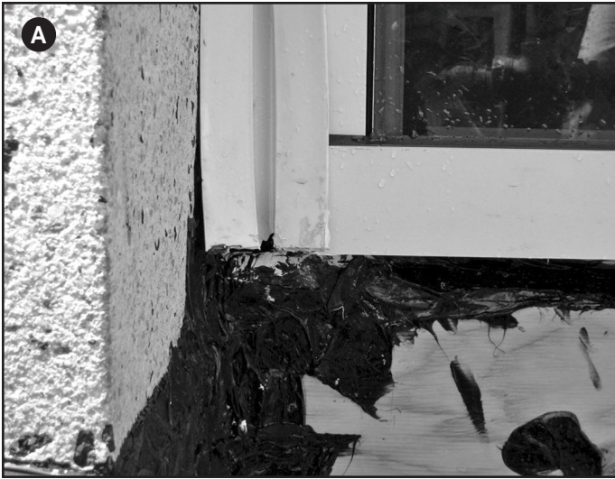
Photo 4A — 2-inch vertical seismic joint between precast concrete panel and curtain wall system. Joint cover system consists of extruded polymeric cover system with integrated bellows attached to aluminum frames (mounting rails). The frames are bedded in sealant on each side and bolted to the adjacent façade systems.; 4B — The interior side of the seismic joint showing the bellows and the frames set in thick beds of sealant. During performance testing, voids in the sealant were discovered, and additional sealant was applied resulting in thick vertical beads of sealant on both sides. The base of the seismic joint consists of a two-piece sheet metal base flashing that is sealed together and onto the wall surface with sealant. Once again, the use of sealant at the base flashing is excessive; and yet, during the first round of testing, the flashing failed.
