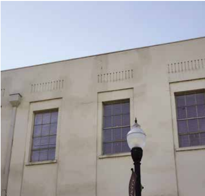
Figure 11. Representative view of cracking in stucco.
