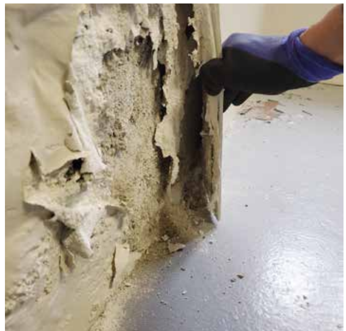
Figure 3. View of low permeability barrier installed at wall interior.
