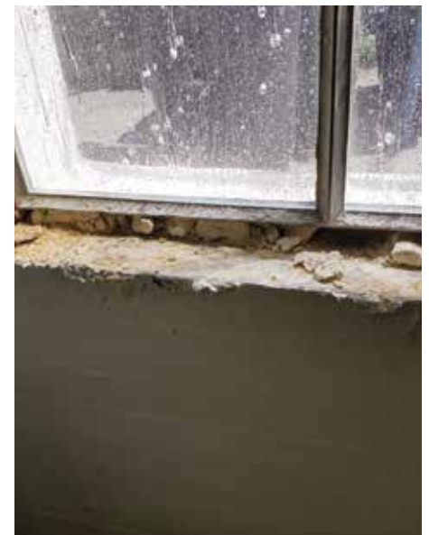
Figure 14. Representative view of soft stucco wrapped into the window rough opening.
