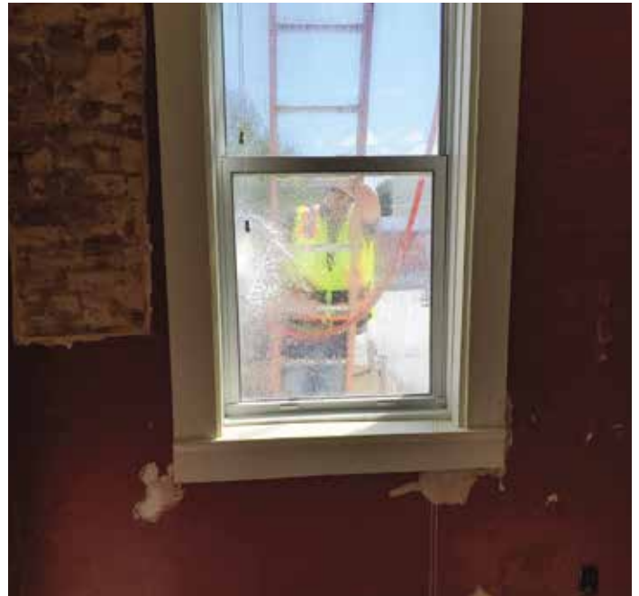
Figure 12. Representative view of forensic water testing.
