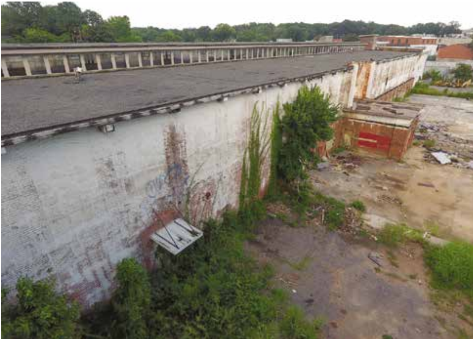
Figure 9. View of cotton mill constructed in 1897.
