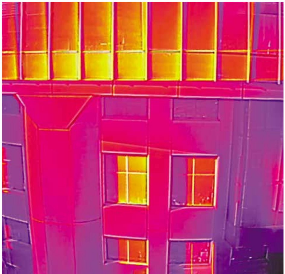
Figure 8. IR facade survey via drone.
