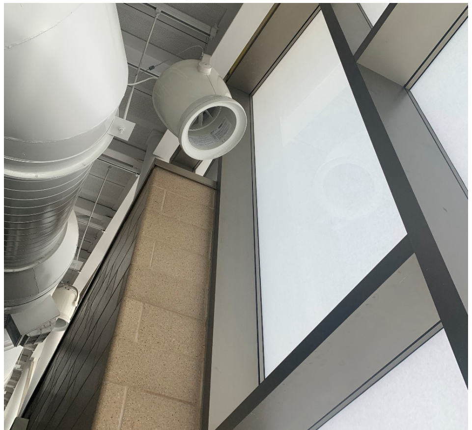
FIGURE 14. Fans were added during the building repairs to blow air directly over the windows to reduce condensation on the interior surfaces of the windows.
