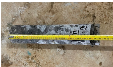
FIGURE 12. Extracted core of foundation wall waterproofing where the membrane was not adhered due to shotcrete overspray.
