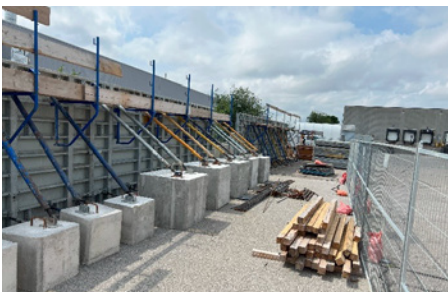
FIGURE 17. UPE Formwork in place for Pouring of Concrete from Bucket.
