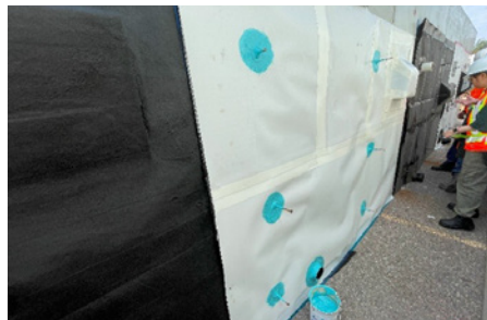
FIGURE 14. High-Density Polyethylene Sheet Waterproofing Installed.
