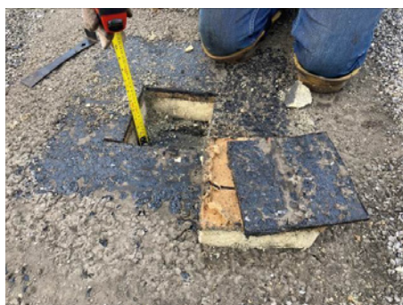
FIGURE 16. Theatre roofs 1993 expansion, plan location, test cut and thermal scan – Pretium Eng. project
