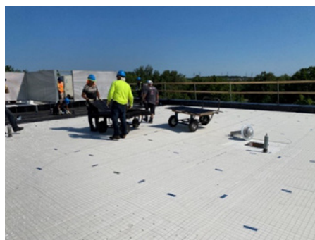
FIGURE 13. Roof assembly installation in progress
