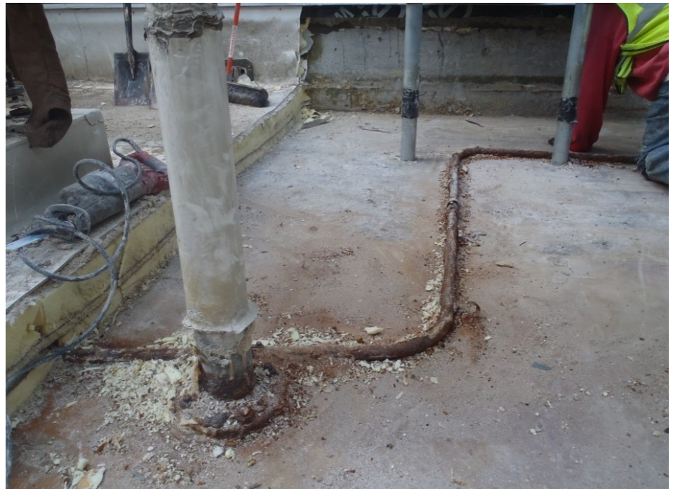
FIGURE 8. Electrical conduit on roof deck within roofing assembly.
