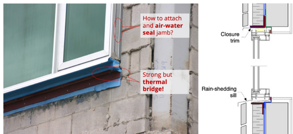
FIGURE 5. Steel angles provide structural support that allow windows to project outward, but impose significant thermal bridging.
