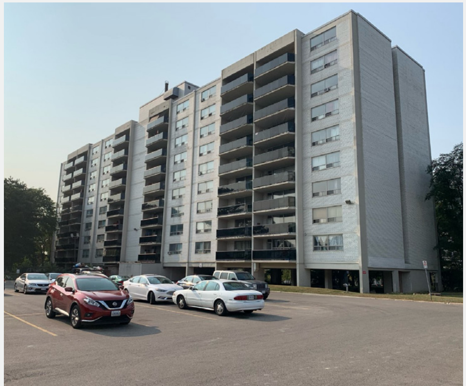
FIGURE 1. East elevation, preconstruction.
