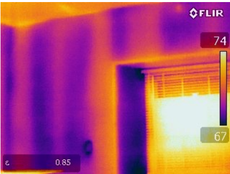
FIGURE 8. Interior infrared image of a historic home and office at a college in Philadelphia, Pennsylvania, originally built 1724.
