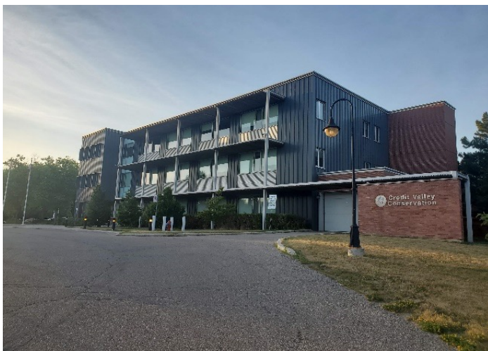
FIGURE 3. CVC Building A - Overview
