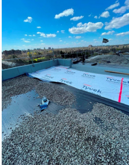
FIGURE 7. New protected membrane roof system under construction.
