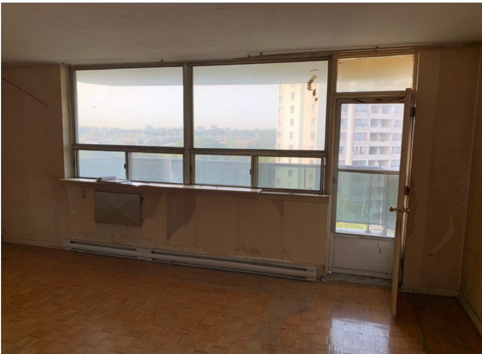
FIGURE 3. Existing in-suite windows and balcony swing doors.
