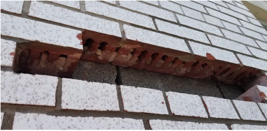
FIGURE 2. Exploratory opening in brick masonry.
