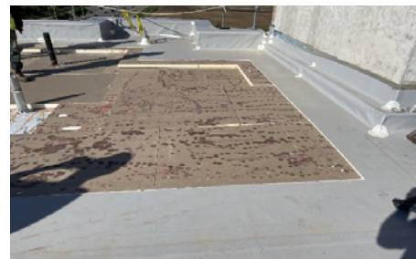
FIGURE 4. Removal of failed roof for repair
