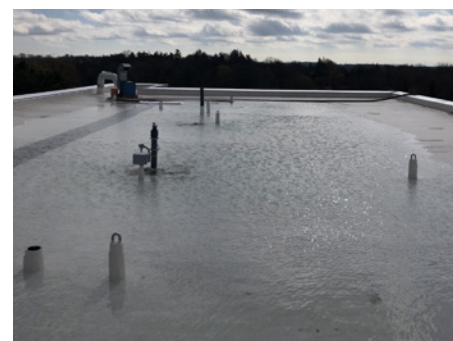
FIGURE 14. Blue roof flood testing in progress
