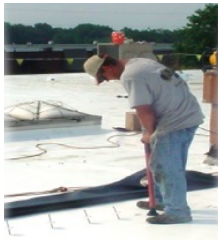
FIGURE 3. TPO roof membrane application – Pretium Eng. project
