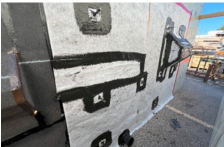
FIGURE 13. UPE Elastomeric Sheet Waterproofing Installed.
