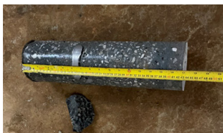
FIGURE 10. Extracted core from foundation wall showing reinforcement bar shadowing.
