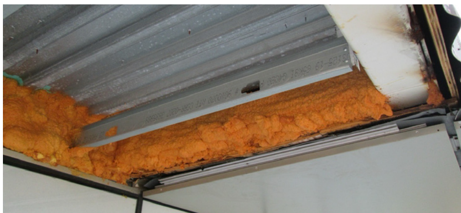
FIGURE 10. Closed-cell spray polyurethane foam (ccSPF) was installed above the windows at the transition between the metal roof deck and the enclosure over the green fluid-applied air and water barrier. ccSPF was also installed around the entire length of the HSS supporting the soffit and connected to the interior structure to minimize thermal bridging.
