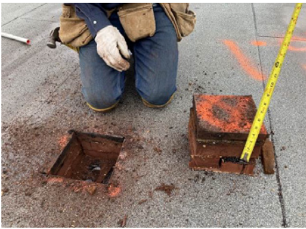
FIGURE 5. Cut tests – Pretium Eng. project
