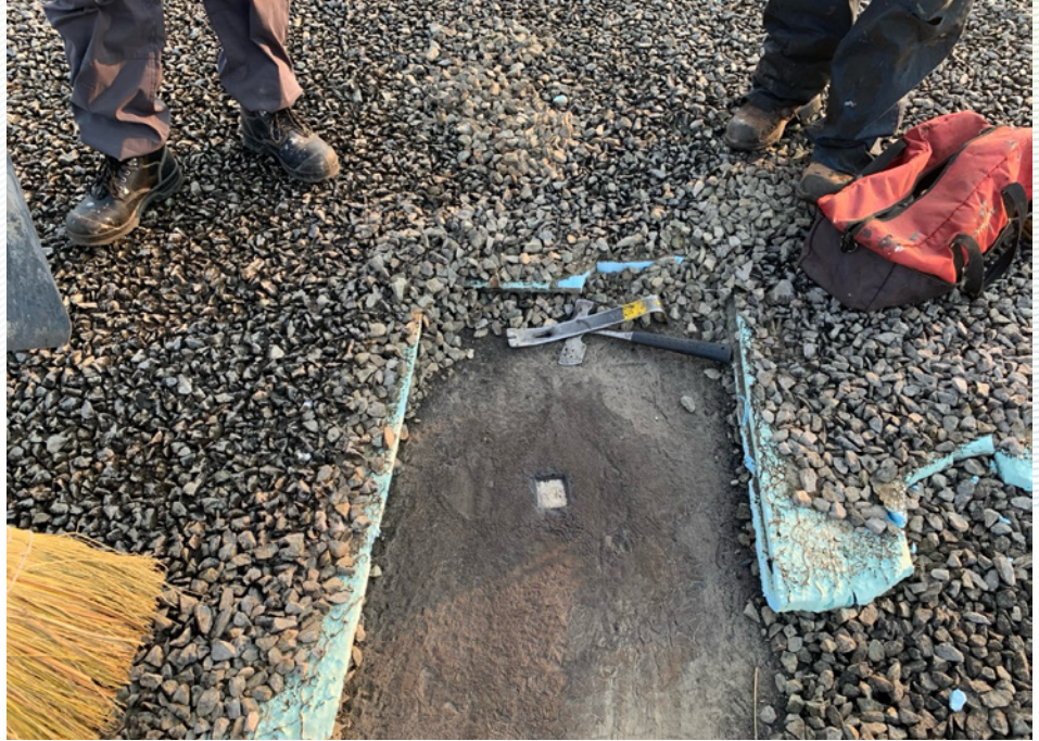
FIGURE 4. Test cut within existing roofing system.
