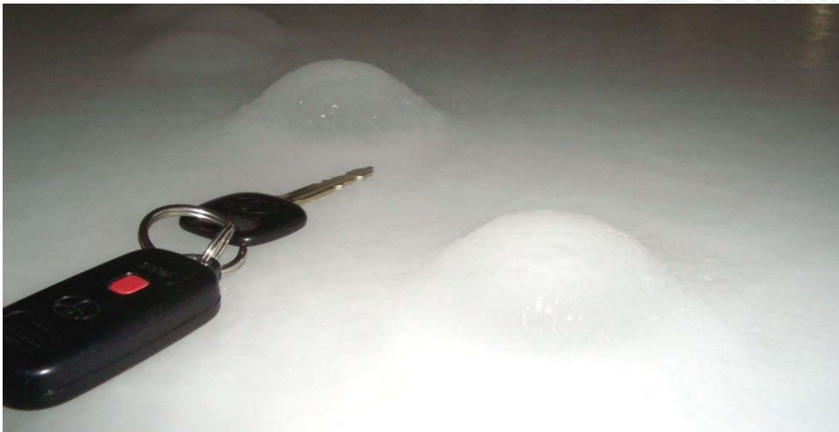
FIGURE 6. Mounding on ice formed when air leaked from the common areas and the pool leaked into the ceiling above the ice rink, condensed, and dripped onto the ice.
