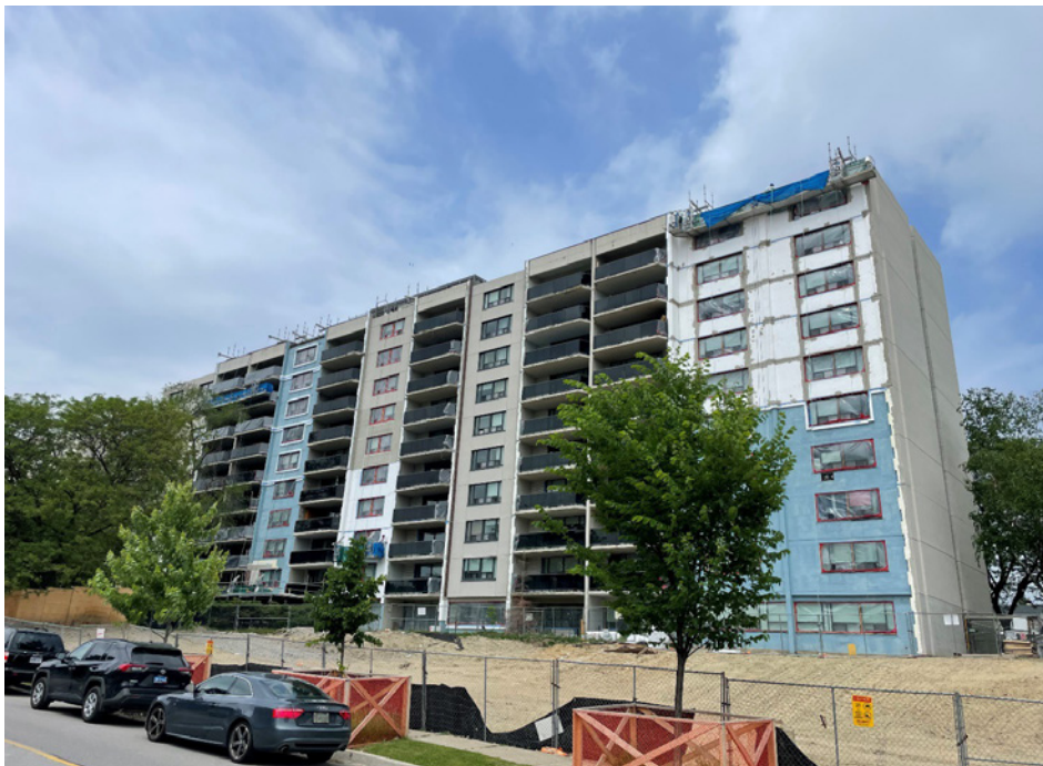
FIGURE 5. Exterior insulation and finish system installation on the west elevation.
