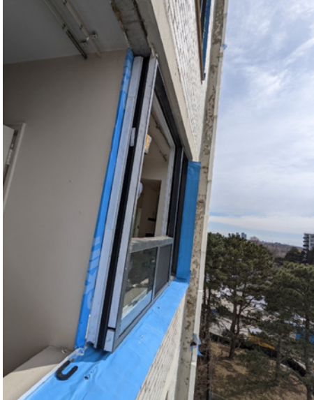
FIGURE 6. New residential window systems with sub-sill flashings.
