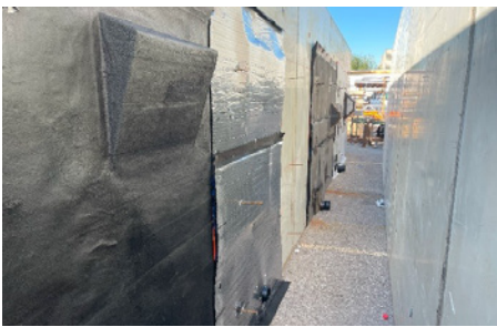
FIGURE 15. UPE Elastomeric Spray Applied Waterproofing Installed.
