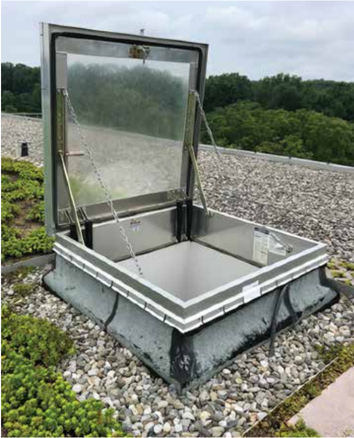
Figure 3. Unprotected non-compliant roof hatch (left photo) versus a OSHA Standard 1910.28 2 -compliant hatch with rails (right photo).
