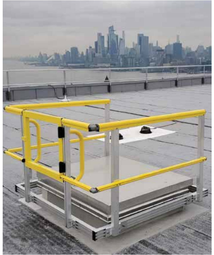
Figure 3. Unprotected non-compliant roof hatch (left photo) versus a OSHA Standard 1910.28 2 -compliant hatch with rails (right photo).
