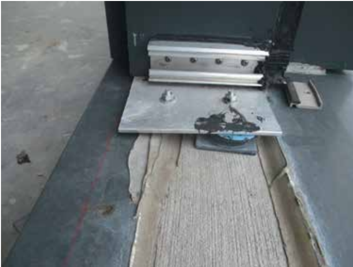
Figure 11. Photo of plastic shims placed under F anchor.
