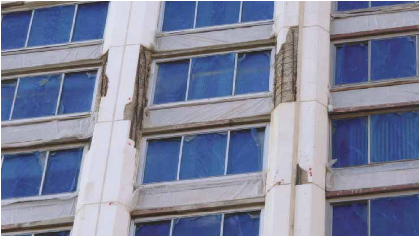
Figure 11. In-progress concrete exterior wall repairs.
