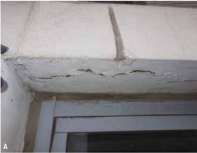
Figure 7. (a) Potentially hazardous delamination and cracking at concrete slab edge soffit; (b) corroded reinforcing steel exposed following removal of spalled concrete.
