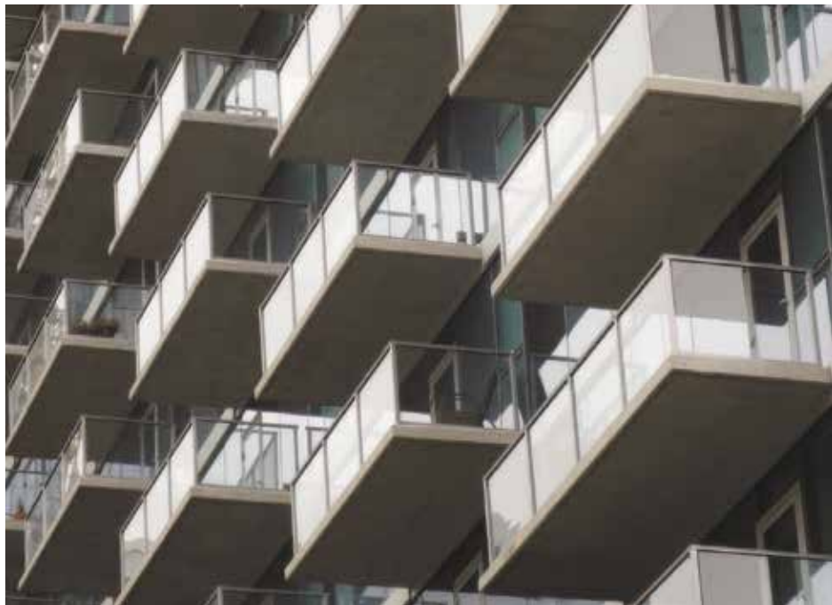
Figure 4. Concrete-frame balconies cantilever beyond the building exterior wall.
