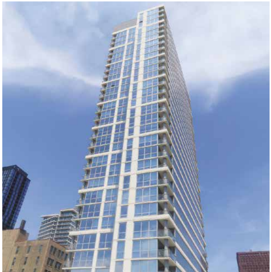
Figure 3. Modern building (circa 2018) with exposed concrete beams, wall areas, columns, slab edges, and balconies.
