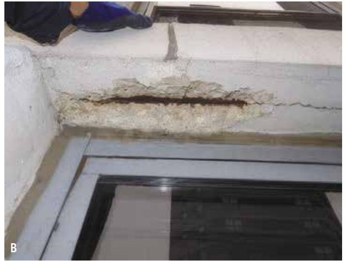
Figure 7. (a) Potentially hazardous delamination and cracking at concrete slab edge soffit; (b) corroded reinforcing steel exposed following removal of spalled concrete.
