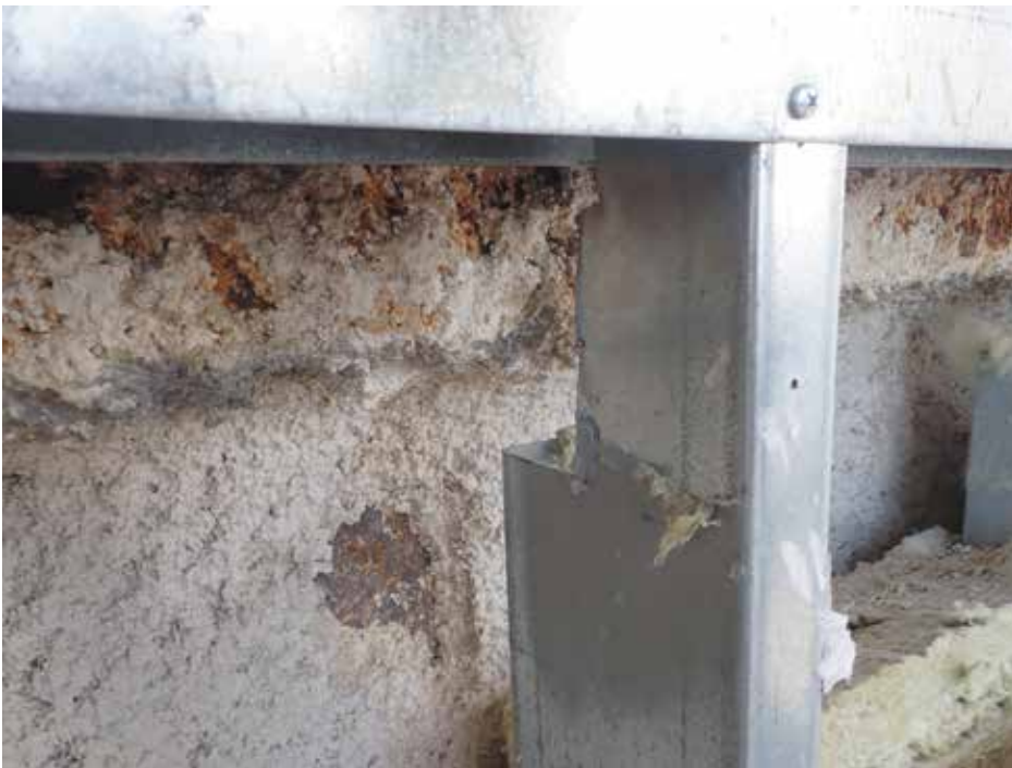
Figure 6. Example of photo documentation of backup wall post-sheathing demolition.
