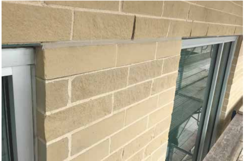
Figure 4. Example of photo documentation of masonry condition pre-masonry demolition.
