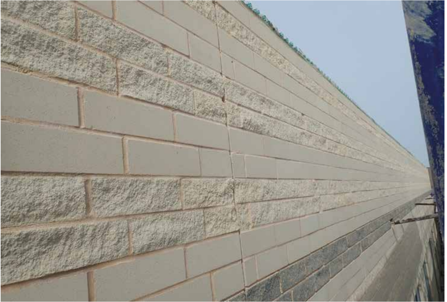
Figure 8. Installation of new masonry units during the reclad construction work.
