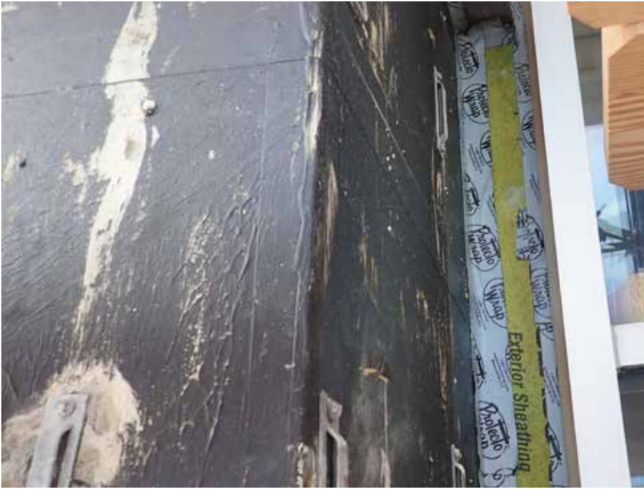
Figure 5. Example of photo documentation of masonry cavity wall post-masonry demolition.
