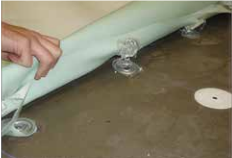
Figure 11. Membrane pullout from the fastener plate in mechanically attached roofing system.
