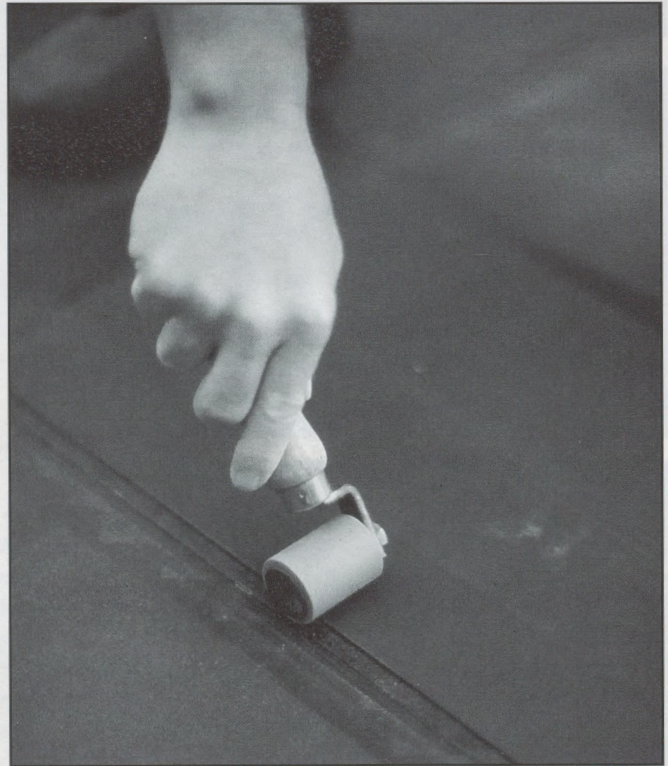
(Clockwise starting with photo to the left) These four photos show taped seams. (1) EPDM seam tapes simplify the seaming process by combining cleaning and priming into one step. (2) When the primer has had sufficient time to flash off (usually less than 10 minutes as verified by the "touch push" test), the tape is applied and rolled in place with a roller to ensure a tight bond with the EPDM. (3) Once the tape is applied, the seam is closed and the release paper is removed. Blooming of the lap promotes "wet-in" of the tape to the primed membrane. (4) The taped seam is finished by hand using a silicone roller to ensure good contact and mating. Taped seams can be installed twice as fast as liquid adhesive seams and offer twice the strength upon aging.
