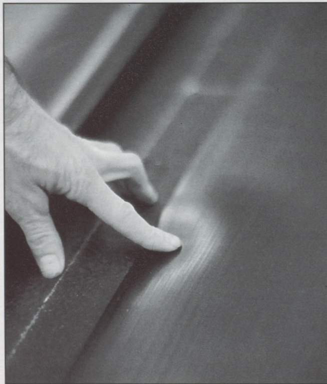
(Clockwise starting with photo to the left) These four photos show taped seams. (1) EPDM seam tapes simplify the seaming process by combining cleaning and priming into one step. (2) When the primer has had sufficient time to flash off (usually less than 10 minutes as verified by the "touch push" test), the tape is applied and rolled in place with a roller to ensure a tight bond with the EPDM. (3) Once the tape is applied, the seam is closed and the release paper is removed. Blooming of the lap promotes "wet-in" of the tape to the primed membrane. (4) The taped seam is finished by hand using a silicone roller to ensure good contact and mating. Taped seams can be installed twice as fast as liquid adhesive seams and offer twice the strength upon aging.
