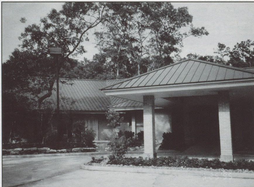
Health facility in Woodlands, Texas. MBCI, Craftsman series standing seam roof was completed in May of 1995. Photos courtesy of Robert Stanford & Associates.
