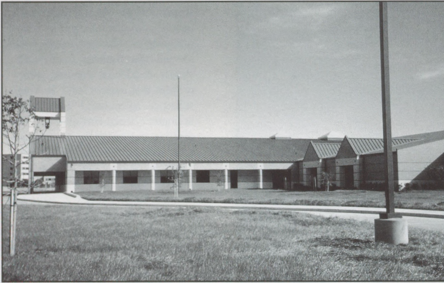
Commercial standing seam roofing system on an elementary school in Alief (Houston area) was completed in November of 1993.
