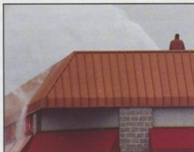
A snow blower will blow snow approximately 20-30 feet. A typical commercial rooftop may be several hundred feet wide. Most of the snow only adds to the load on an adjacent section of the roof.
